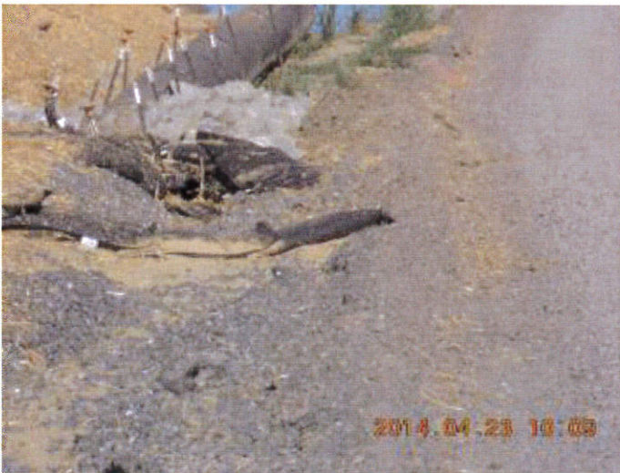
Photo 27: West side of U2 line, looking north toward the storm water basin shown in Photo 26. An attempt had been made to intercept drainage from the ditch shown in Photo 26, by installing the smaller black plastic pipe, but storm water scoured beneath the pipe and eroded the earthen ditch immediately downstream.
