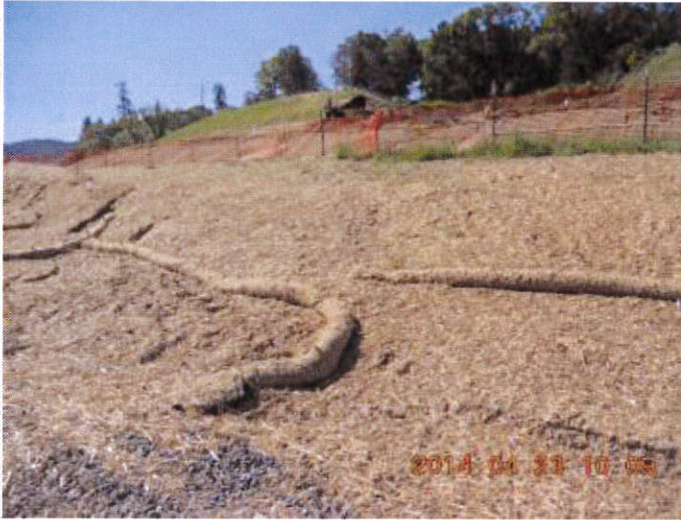
Photo 23: Just north of the basin shown in Photo 21. Erosion from uncontrolled run-on.
