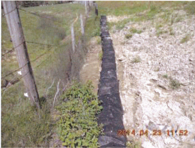
Photo 57: Looking north. Erosion and sediment transport and discharge off-site at the toe of slope along the U3 line. The contractor's Water Pollution Control Manager discussed plans to remove sediment and install erosion control fabric and gravel bag check dams within the channel. I do not know exactly where this off-site drainage discharges.
