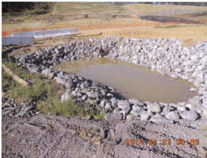
Photo 21. Looking west at Hwy 101. This basin receives all flow from the basin shown in Photo 12 and discharges into the drainage system shown in Photo 27. This basin is eroding as seen in the top left of the photo, just to the left of the rock-slope protection. This basin must be stabilized.
