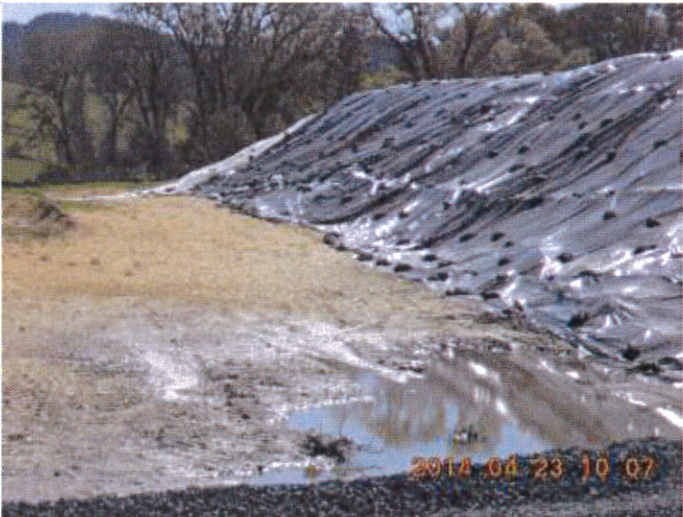
Photo 55: This basin primarily drains to Basin 1 through an inlet just to the lower right of the photo (see Photo 56), but will overflow directly to South Haehl Creek at the location in the upper left of the photo and as shown in Photo 54.
