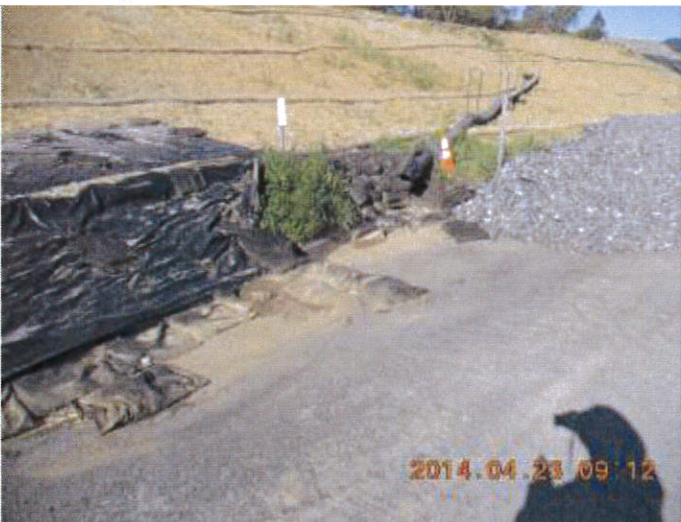
Photo 13: The basin shown in Photo 12 discharges to this drainage inlet on Hwy 101 before being carried under the highway to the basin shown in Photo 21
