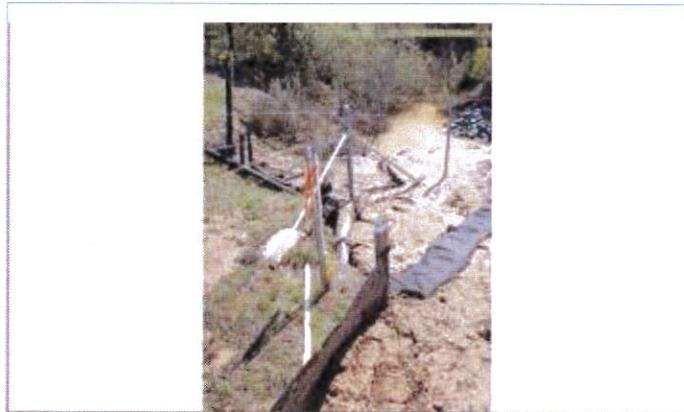
Photo 42. Looking southeast at Drainage System 24 before it enters a culvert and discharges to South Haehl Creek. A large gully has formed developed into the channel, as seen in the center of the photo. The steel fence is the Caltrans right-of-way fence. Caltrans staff said they were limited to fixes within their right-of-way; however, the disturbance on the other side of the fence was created by Caltrans and is Caltrans's responsibility to stabilize.
