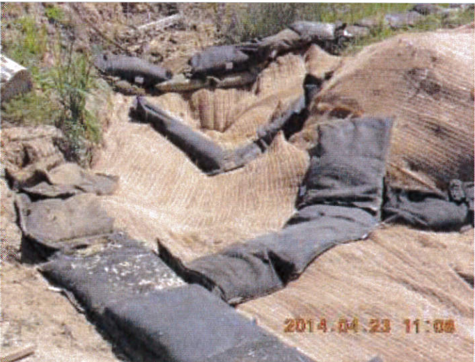
Photo 45: A closer view of the area shown in Photo 44, upper right. This watercourse runs into Caltrans's project limits from the Schmidbauer property, just before discharging to South Haehl Creek. Because a stable drainage path to South Haehl Creek was not planned for and provided, drainage has eroded the creek bank and transported sediment to South Haehl Creek. A stable drainage path must be provided. Plans for the final drainage configuration must be approved by the Regional Water Board. Biotechnical elements should be incorporated as appropriate.
