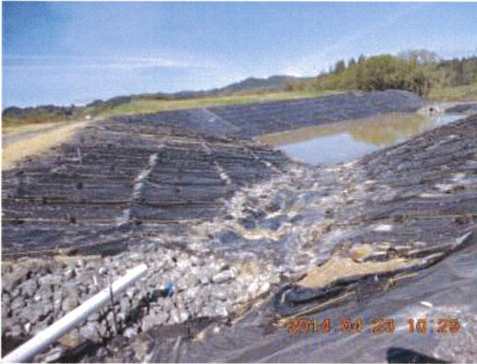
Photo 31: A view of Basin 1, looking north. The channel was eroding/eroded below the outlet seen in the foreground. This channel must be appropriately stabilized to accommodate concentrated flow.
