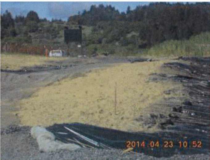
Photo 33: At the top of Basin 1, southern side, looking west. This dirt area was unstabilized and eroding. This area and others around the basin must be stabilized.
