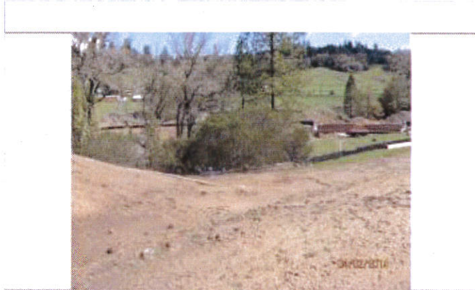
Photo 54: There was evidence that the basin shown in Photo 19 and Photo 55 overflowed down this slope, through the silt fence, and into South Haehl Creek. Erosion can be seen in the center-right of the photo. The silt fence shown in the distance was worn and requires replacement.
