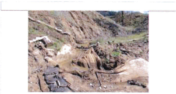
Photo 45: A closer view of the area shown in Photo 44, upper right. This watercourse runs into Caltrans's project limits from the Schmidbauer property, just before discharging to South Haehl Creek. Because a stable drainage path to South Haehl Creek was not planned for and provided, drainage has eroded the creek bank and transported sediment to South Haehl Creek. A stable drainage path must be provided. Plans for the final drainage configuration must be approved by the Regional Water Board. Biotechnical elements should be incorporated as appropriate.
