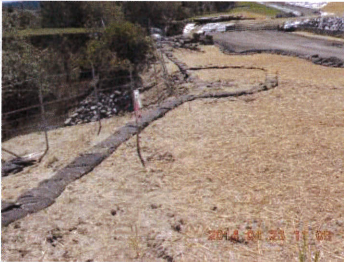
Photo 41 Looking south at Drainage System 24 before it enters a culvert and discharges to South Haehi Creek. There was inadequate erosion and sediment control in this area. This area must be stabilized.
