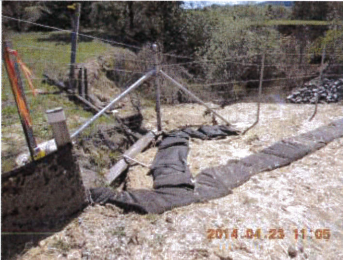
Photo 42. Looking southeast at Drainage System 24 before it enters a culvert and discharges to South Haehl Creek. A large gully has formed developed into the channel, as seen in the center of the photo. The steel fence is the Caltrans right-of-way fence. Caltrans staff said they were limited to fixes within their right-of-way; however, the disturbance on the other side of the fence was created by Caltrans and is Caltrans's responsibility to stabilize.
