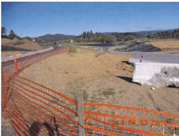
Photo 22: This area is just south of the main entrance-way to Area 1 and between the existing Hwy 101 and the basin shown in Photo 21. This area is without and requires erosion and sediment control. Photo 23 shows erosive conditions resulting from this uncontrolled run-on.
