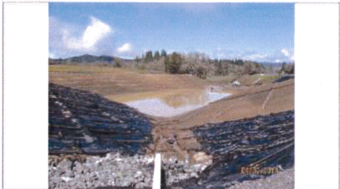
Photo 31: A view of Basin 1, looking north. The channel was eroding/eroded below the outlet seen in the foreground. This channel must be appropriately stabilized to accommodate concentrated flow.
