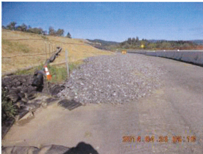
Photo 16. Looking north along the shoulder of Hwy 101 where gravel was placed as a sediment control. The road slopes downward and the gravel extends to the location of a drain inlet (see Photo 17) that transports stormwater under the free-way to the basin shown in Photo 28.
