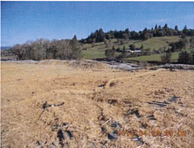
Photo 24: Looking northeast at the "U2" fill area, just east of main entrance to Area 2. Sediment transport was evident throughout the area despite the recently placed straw erosion control.
