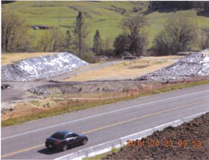
Photo 19: A view across the highway, looking east, at two more areas where stormwater is stored before discharging to South Haehl Creek. The basin in the foreground discharges to Basin 1 and the one in the background discharges to both the basin in Photo 18 and during periods of overflow directly into South Haehl Creek as described in Photo 54
