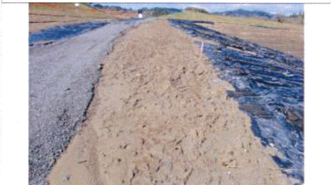
Photo 33: At the top of Basin 1, southern side, looking west. This dirt area was unstabilized and eroding. This area and others around the basin must be stabilized.
