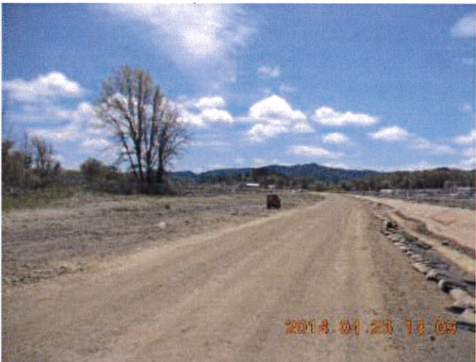
Photo 62: Looking south at disturbed area south of Bent 1. This large area has generally inadequate erosion and sediment controls. This area discharges to a tributary of Beechdale Creek at the location shown in Photo 63.
