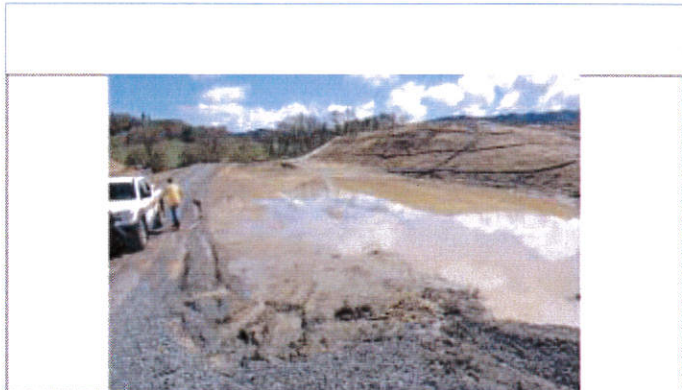
Photo 55: This basin primarily drains to Basin 1 through an inlet just to the lower right of the photo (see Photo 56), but will overflow directly to South Haehl Creek at the location in the upper left of the photo and as shown in Photo 54.
