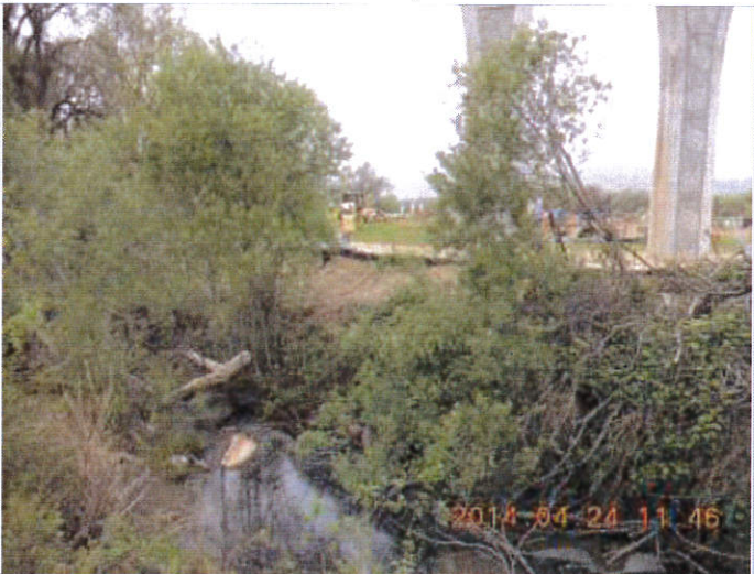
Photo 72: Looking north-west. Sediment discharge to Baechtel Creek at Pier 4 as a result of inadequate erosion control and failed sediment control. Erosion and sediment control must be provided.
