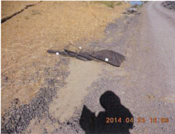
Photo 26: Looking north on the U2 line toward the basin shown in Photo 27 and Photo 28. Sediment had inundated this check dam during the previous rain event and gullying occurred downstream as a result.
