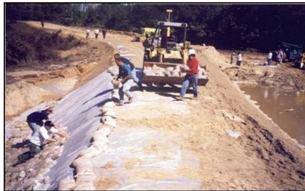
Figure 1.6: Levee Repair after Hurricane Floyd, 2000
