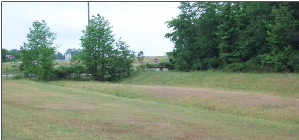
Figure 2.8: Southern End of Levee
