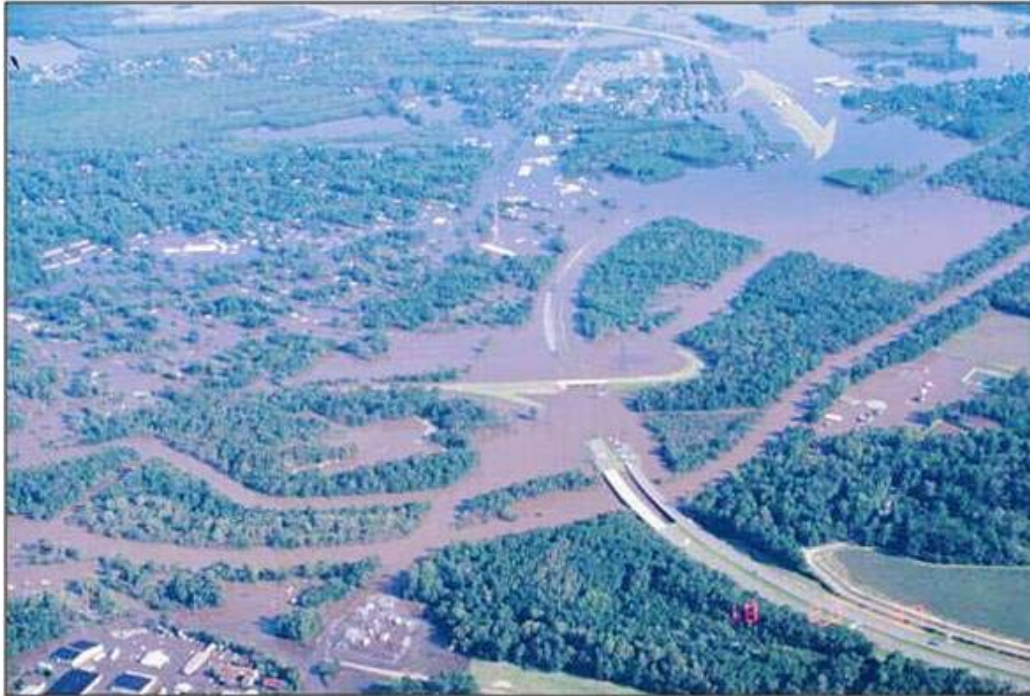
Figure 1.3: Hurricane Floyd Flooding, September 1999 (view from Northeast)
