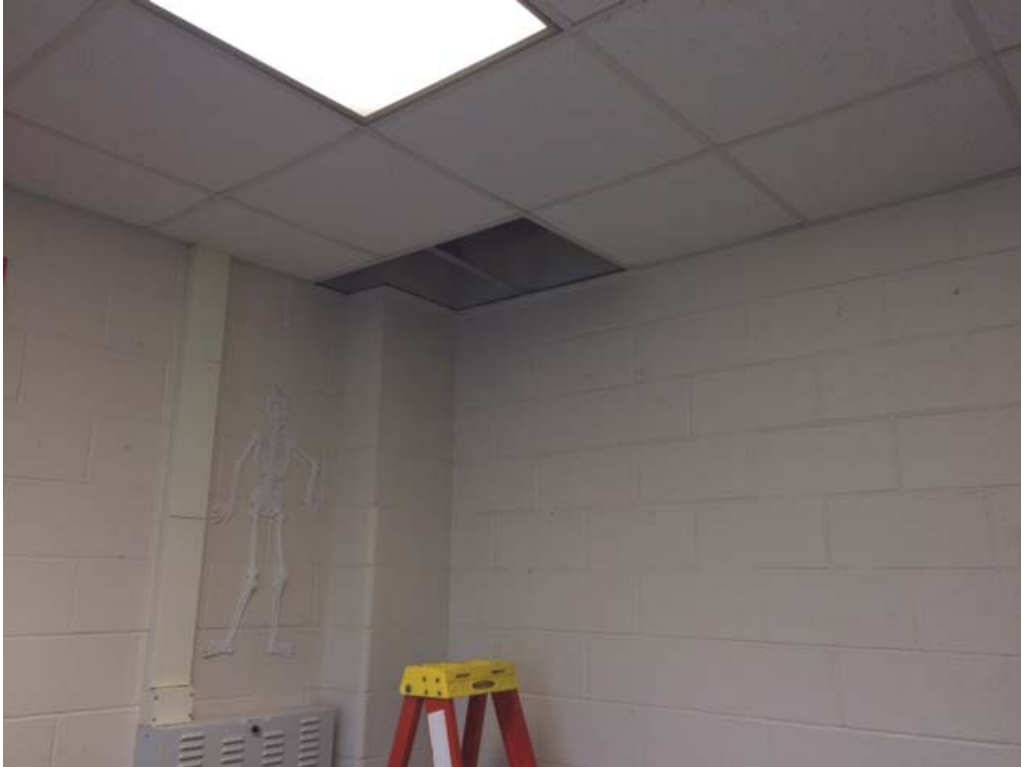
Target area of investigation in classroom 3320.
