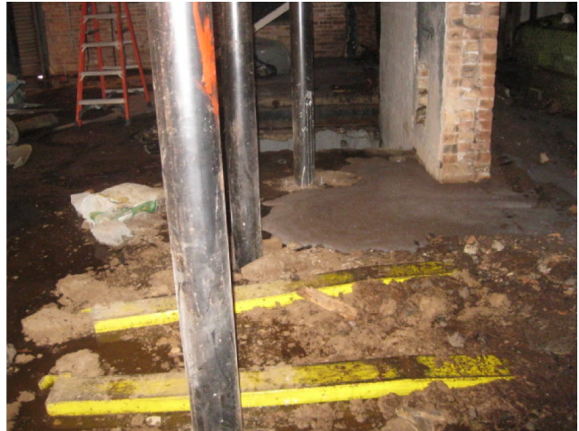
Date: 12/14/2015 5:49 AM Description: STRUCTURAL WORK WITHOUT PLANS & PERMITS
