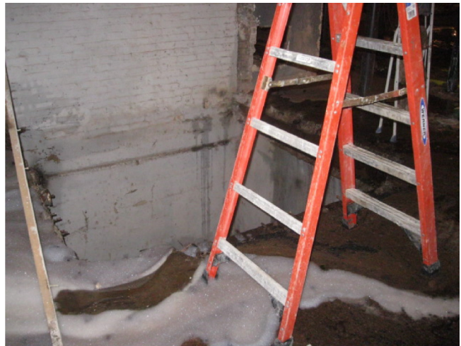
Date: 12/14/2015 5:49 AM Description: ELEVATOR SHAFT W/ OPEN FLOOR
