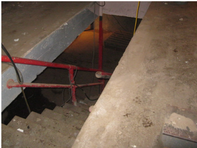
Date: 12/14/2015 5:49 AM Description: STAIR SYSTEM WITH MISSING HANDRAILS
