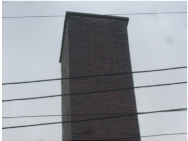
Date: 12/14/2015 5:49 AM Description: CHIMNEY AT NORTH ELEVATION
