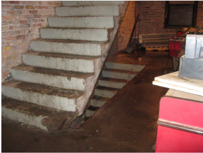
Date: 12/14/2015 5:49 AM Description: MISSING GUARD & HANDRAILS
