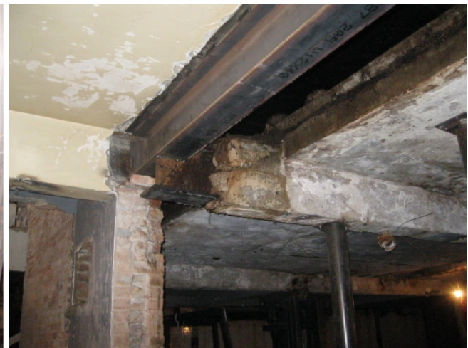
Date: 12/14/2015 5:49 AM Description: STRUCTURAL WORK WITHOUT PLANS &
