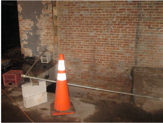
Date: 12/14/2015 5:49 AM Description: OPEN ELEVATOR SHAFT
