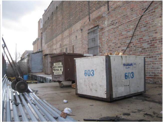
Date: 12/14/2015 5:49 AM Description: EAST ELEVATION
