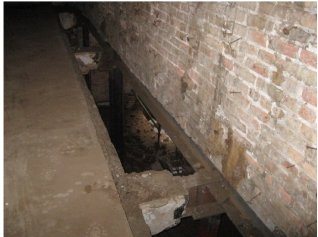
Date: 12/14/2015 5:49 AM Description: OPENINGS AT 2ND FLOOR INTERIOR WALL
