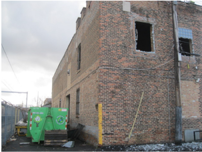
Date: 12/14/2015 5:49 AM Description: EAST ELEVATION
