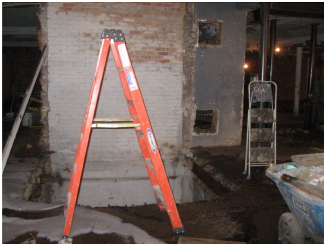
Date: 12/14/2015 5:49 AM Description: DEMOLISHED ELEVATOR SHAFT W/ OPEN FLOOR
