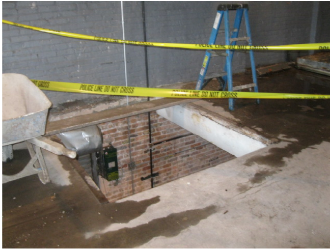
Date: 12/14/2015 5:49 AM Description: OPEN ELEVATOR SHAFT
