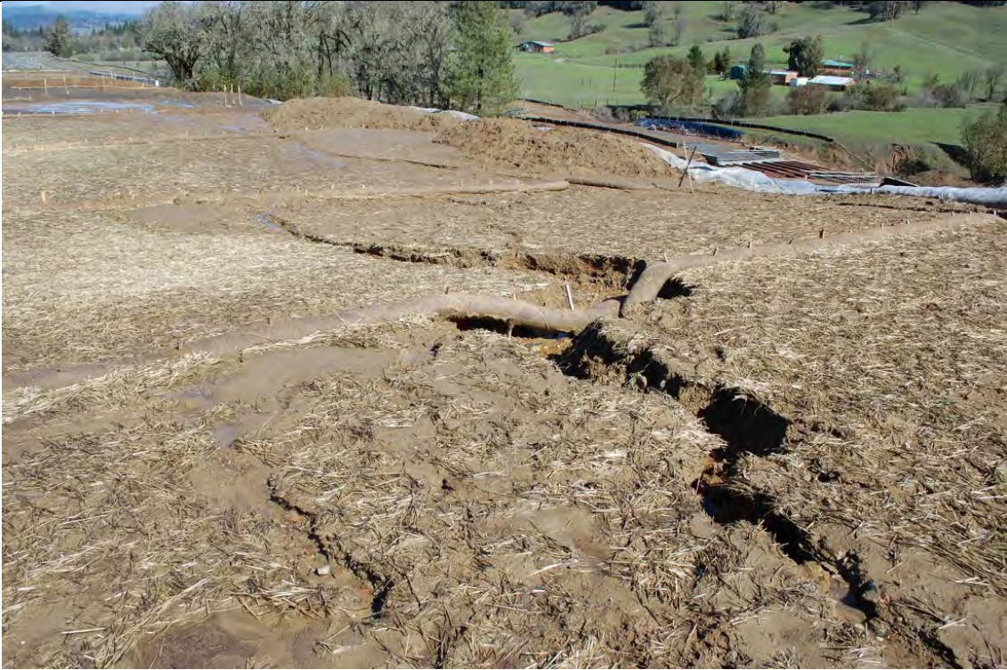
Photo 24: Looking northeast at the “U2” fill area, just east of main entrance to Area 2. Sediment transport was evident throughout the area despite the recently placed straw erosion control.
