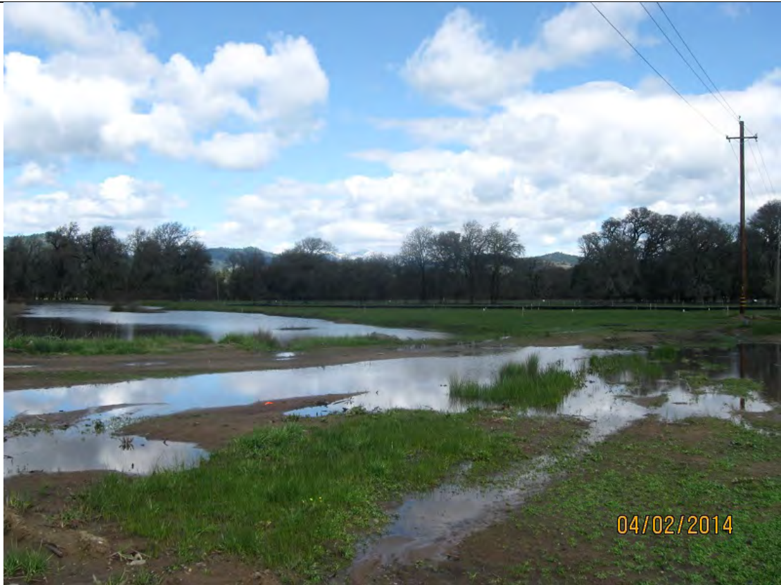
Photo 68: Looking northeast at Rutledge Pond. No sediment control at the boundary of Rutledge Pond. Construction storm water has flowed uncontrolled into the pond all rainy season. Perimeter control must be installed.
