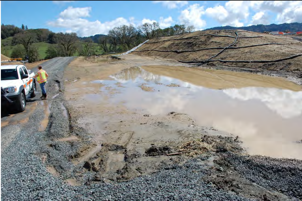
Photo 55: This basin primarily drains to Basin 1 through an inlet just to the lower right of the photo (see Photo 56), but will overflow directly to South Haehl Creek at the location in the upper left of the photo and as shown in Photo 54.
