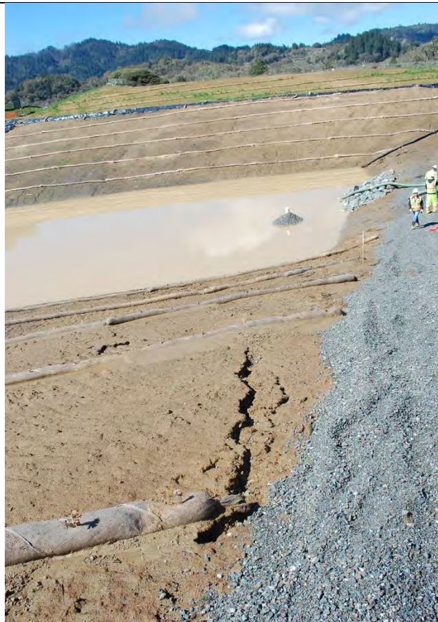
Photo 35: At the top of Basin 1, northern side, looking west. This dirt area, and the area immediately to the south at the top of the basin was unstabilized and eroding. These areas must be stabilized.
