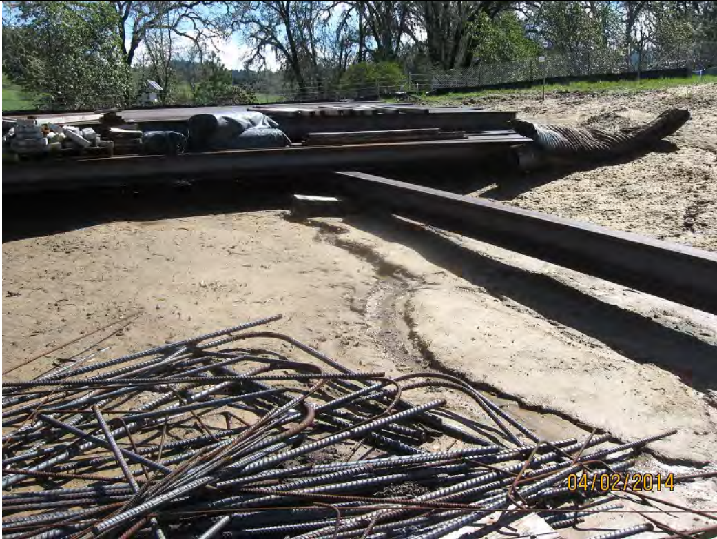
Photo 48: Looking east at a material storage area, just south of South Haehl Creek at the bridge 0129 abutment. Inadequate erosion and sediment controls. The eroding channel flows toward south Haehl Creek.
