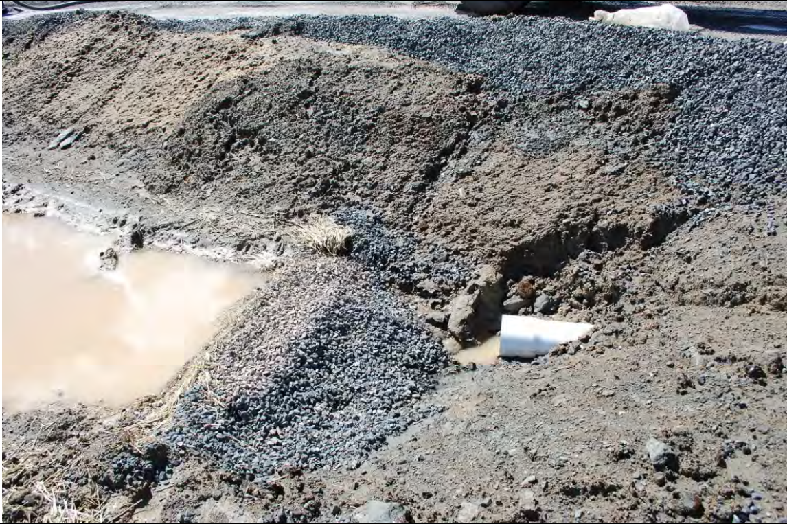
Photo 56: The outlet of the basin shown in Photo 55. A gravel bar has been added before the outlet for sediment filtration.
