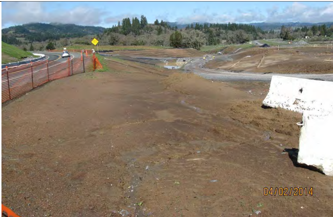
Photo 22: This area is just south of the main entrance-way to Area 1 and between the existing Hwy 101 and the basin shown in Photo 21. This area is without and requires erosion and sediment control. Photo 23 shows erosive conditions resulting from this uncontrolled run-on.
