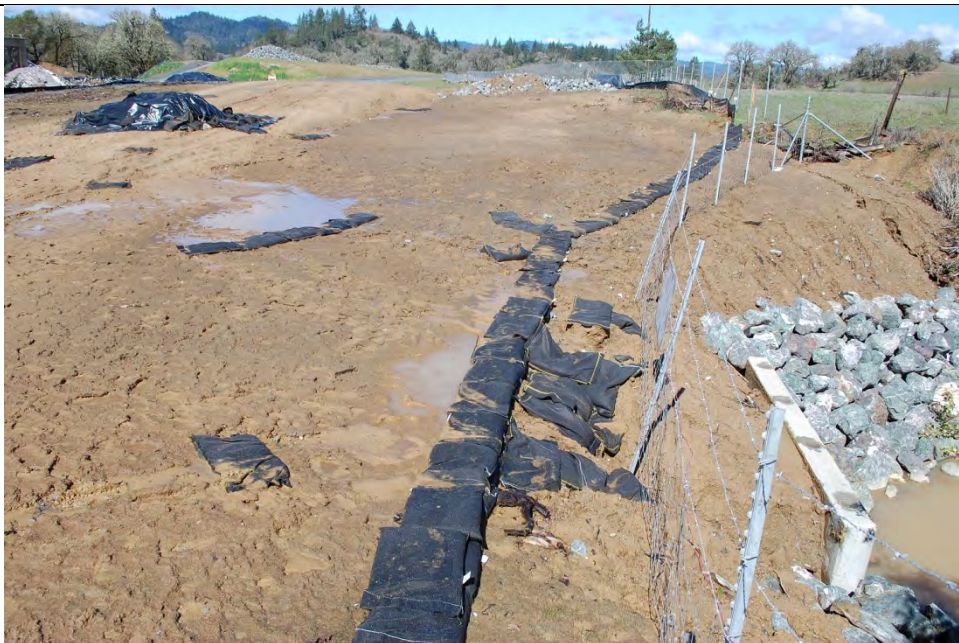
Photo 43: Looking north at Drainage System 24.
