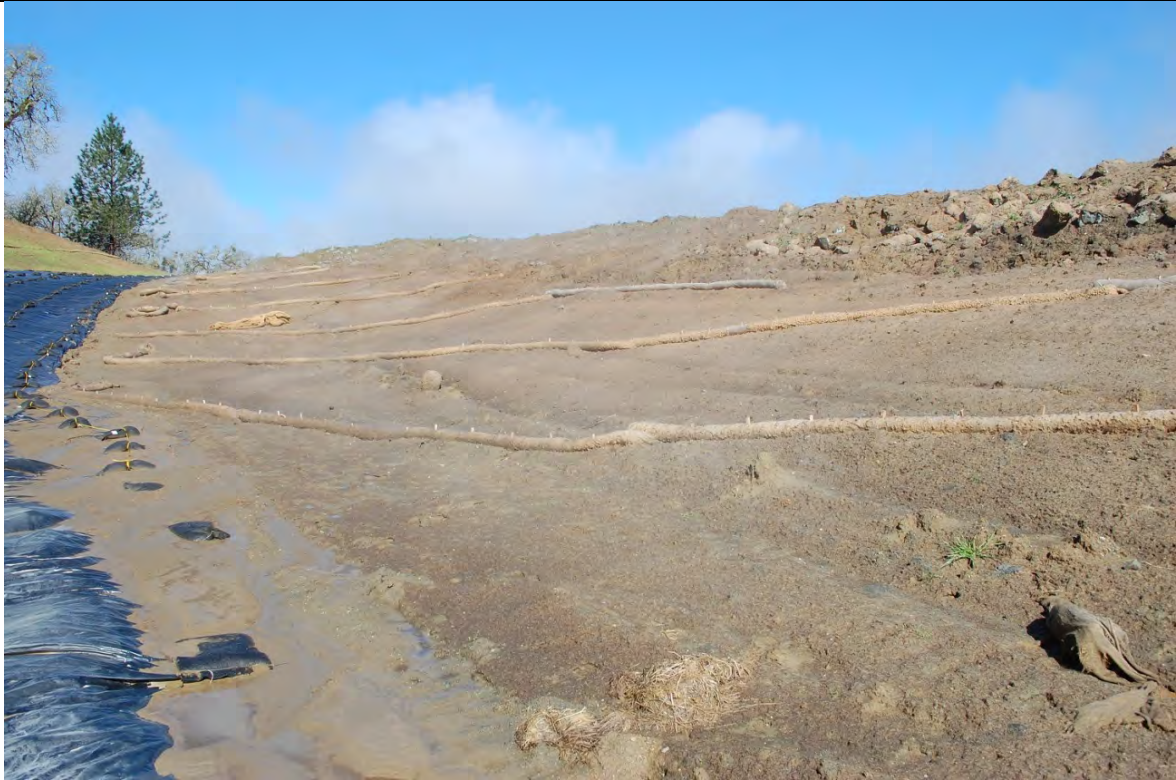
Photo 14: Part of a rock and dirt stockpile approximately across from the area shown in Photo 11. Runoff from the plastic sheeting was causing erosion adjacent the edge of the sheeting.
