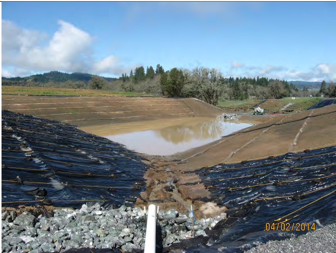
Photo 31: A view of Basin 1, looking north. The channel was eroding/eroded below the outlet seen in the foreground. This channel must be appropriately stabilized to accommodate concentrated flow.
