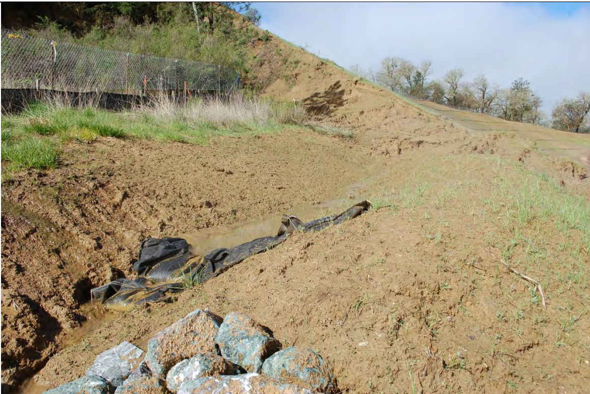
Photo 5: Top of disturbed slope shown in Photo 4. Only one gravel bag check dam and no effective erosion control was present. The rock in the bottom of the picture is the top of the rock-lined drainage ditch shown in Photo 4.
