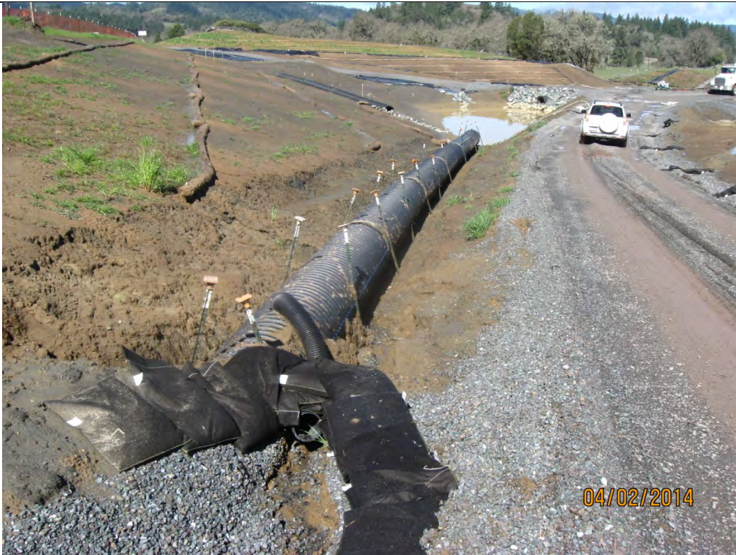
Photo 27: West side of U2 line, looking north toward the storm water basin shown in Photo 26. An attempt had been made to intercept drainage from the ditch shown in Photo 26, by installing the smaller black plastic pipe, but storm water scoured beneath the pipe and eroded the earthen ditch immediately downstream.
