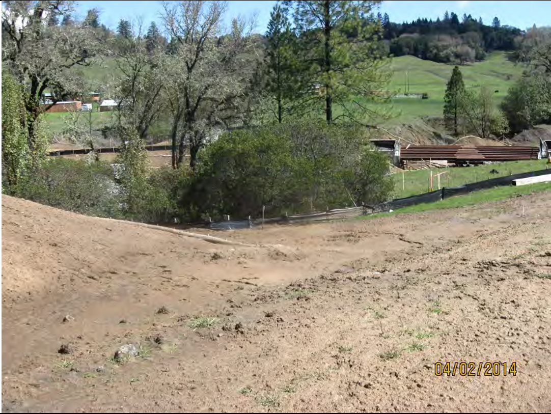
Photo 54: There was evidence that the basin shown in Photo 19 and Photo 55 overflowed down this slope, through the silt fence, and into South Haehl Creek. Erosion can be seen in the center-right of the photo. The silt fence shown in the distance was worn and requires replacement.
