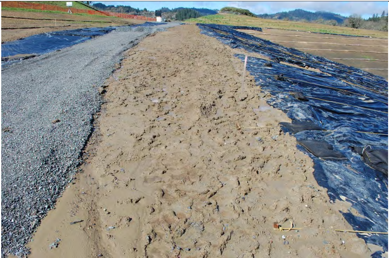
Photo 33: At the top of Basin 1, southern side, looking west. This dirt area was unstabilized and eroding. This area and others around the basin must be stabilized.
