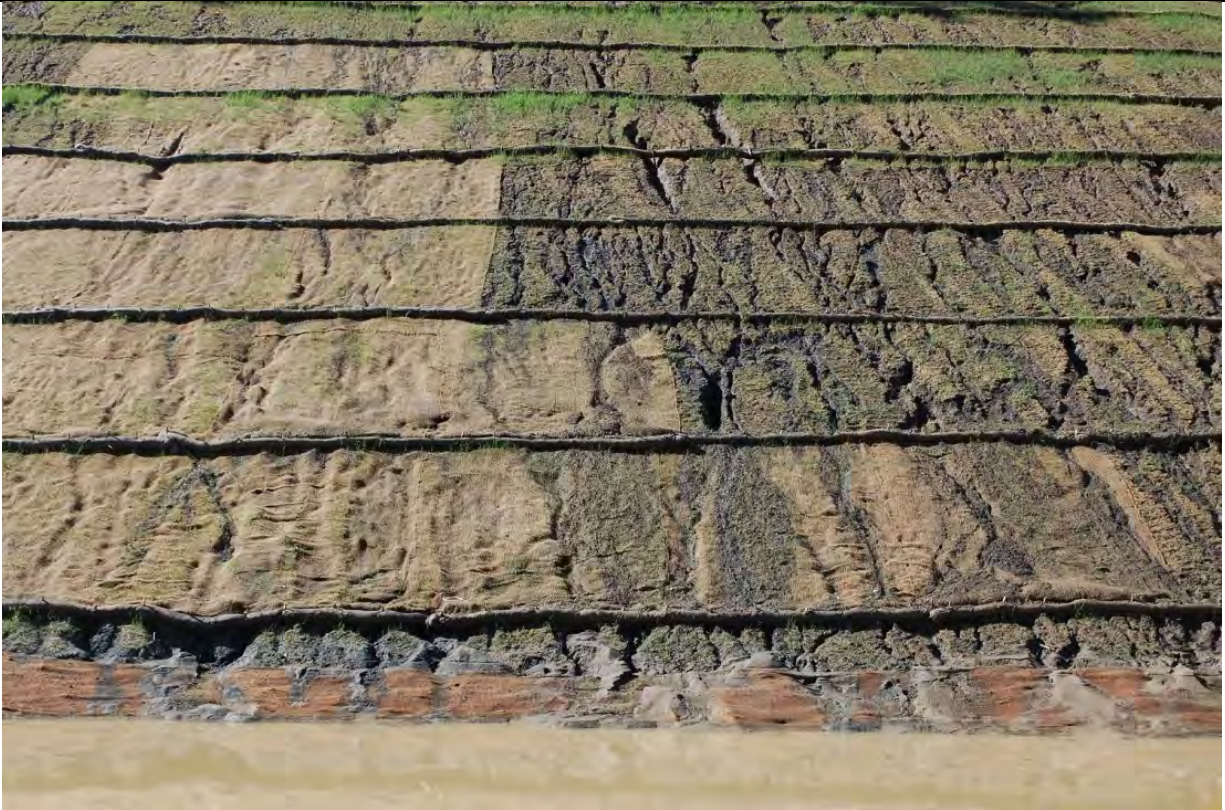
Photo 10: A close-up of gullying on the slope shown in Photo 9, with the storm water basin below.
