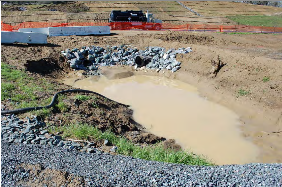
Photo 21: Looking west at Hwy 101. This basin receives all flow from the basin shown in Photo 12 and discharges into the drainage system shown in Photo 27. This basin is eroding as seen in the top left of the photo, just to the left of the rock-slope protection. This basin must be stabilized.
