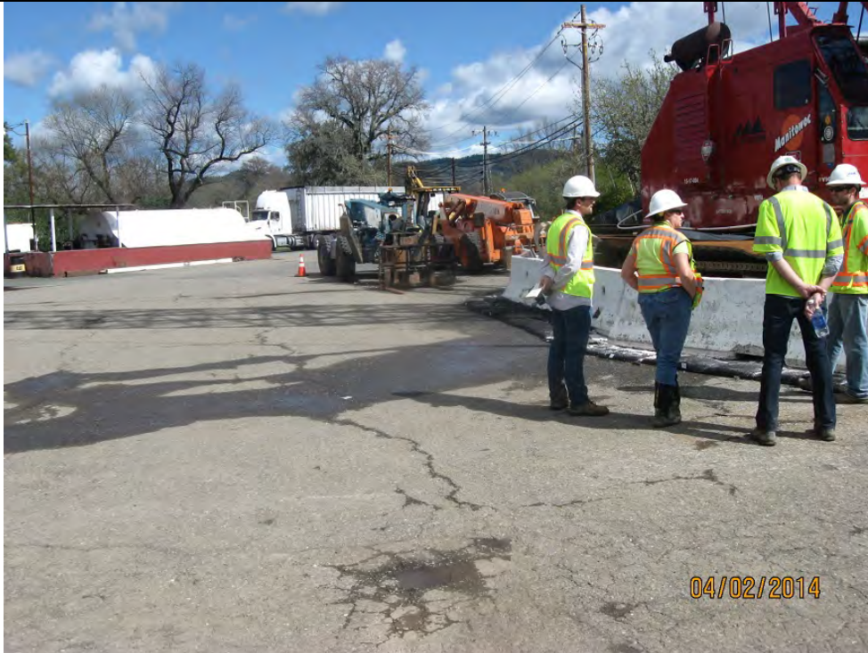
Photo 71: It appeared that fluid had drained from the spill area as indicated by the water mark on the asphalt. We communicated that the material, including the gravel bags must be disposed of immediately, subject to appropriate hazardous waste disposal protocol. Caltrans had not been notified of the incident and potential discharge.
