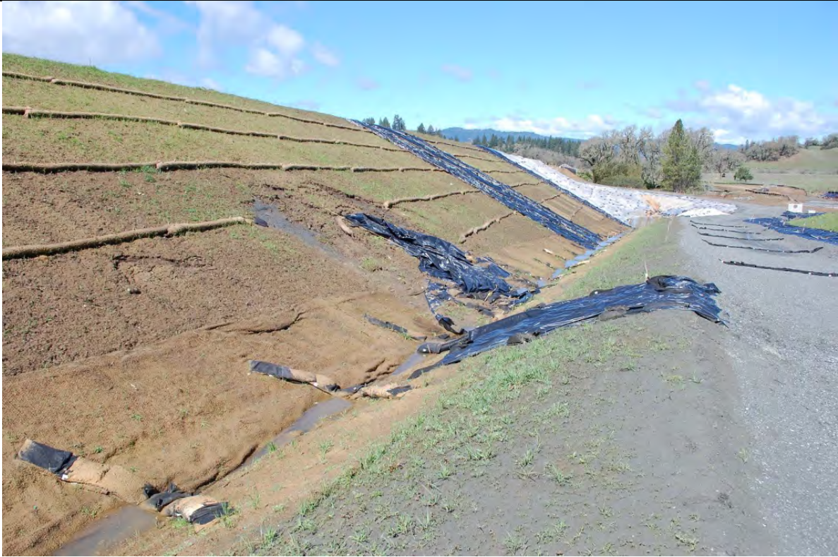
Photo 50: Drainage ditch on the west side of the U2 line, looking north. Ditch incision and sediment transport was evident in several locations.
