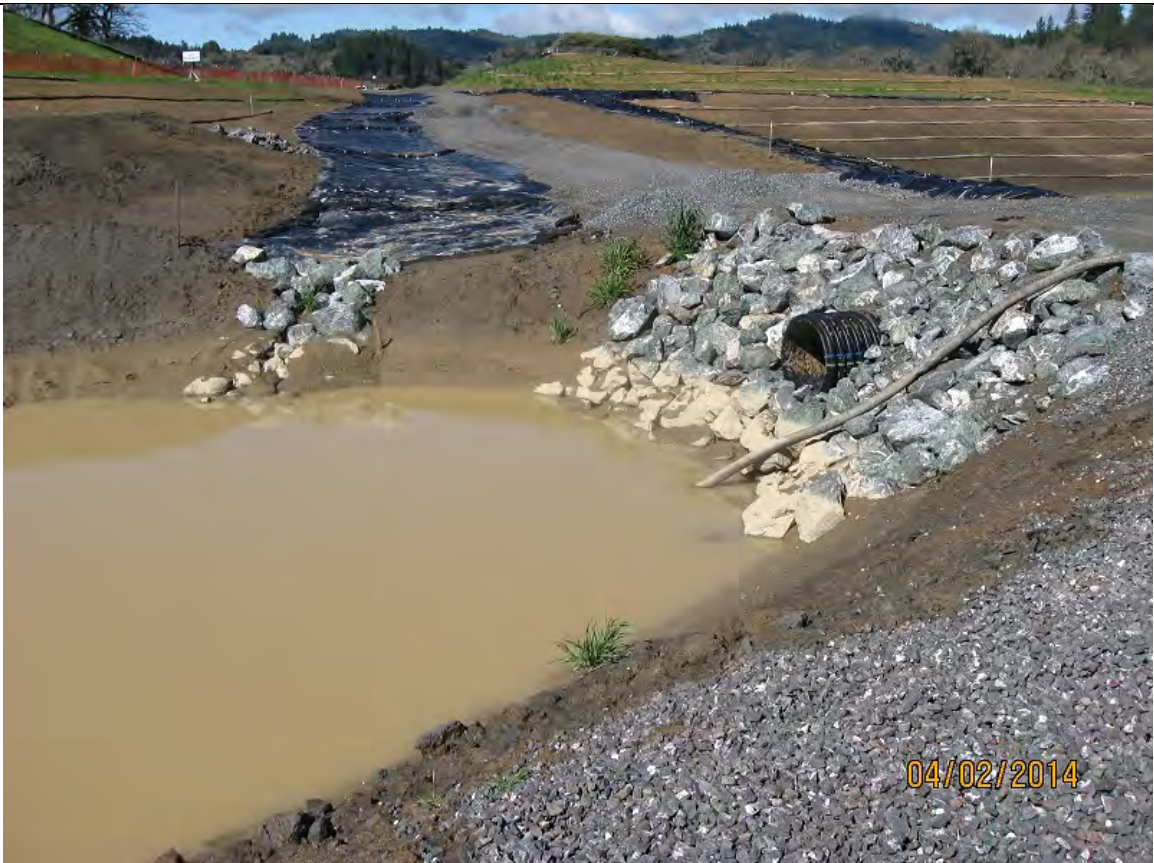
Photo 29: The outlet of the basin shown in Photo 28.
