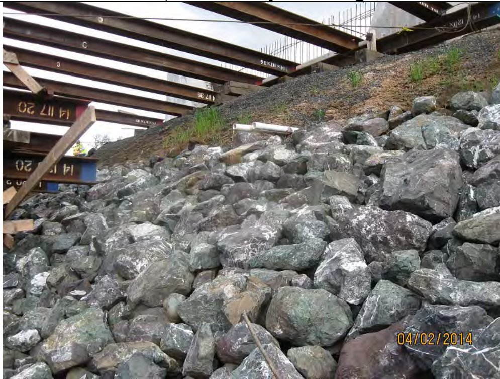
Photo 60: Discharge of high pH water from the North Haehl Creek southern abutment. High pH water had been discharging for an unknown period of time as a result of storm water infiltration through concrete base aggregate. The pipe has since been capped to prevent discharge.
