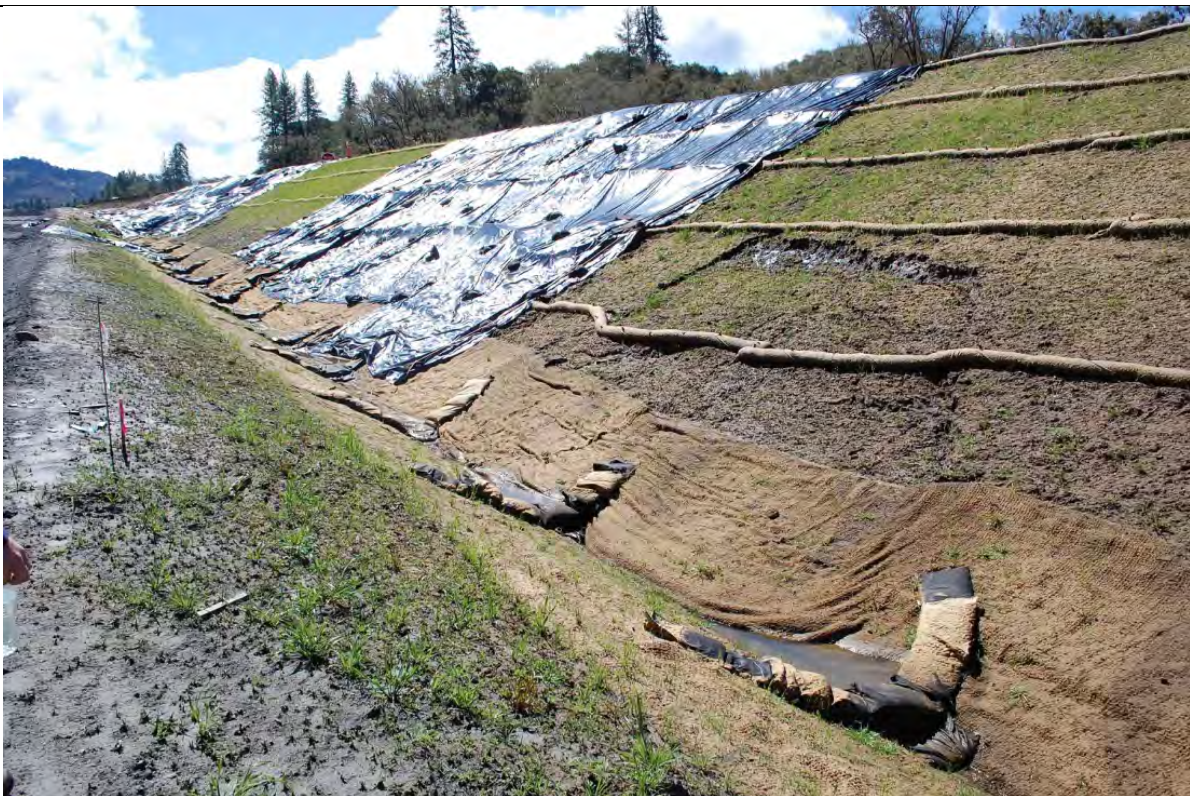
Photo 49: Drainage ditch on the west side of the U2 line, looking south. The slope was failing and eroding in several locations. Some of the slides are restricted to the top six inches, which corresponds to the depth of compost incorporation. This area drains to the basin shown in Photo 25.
