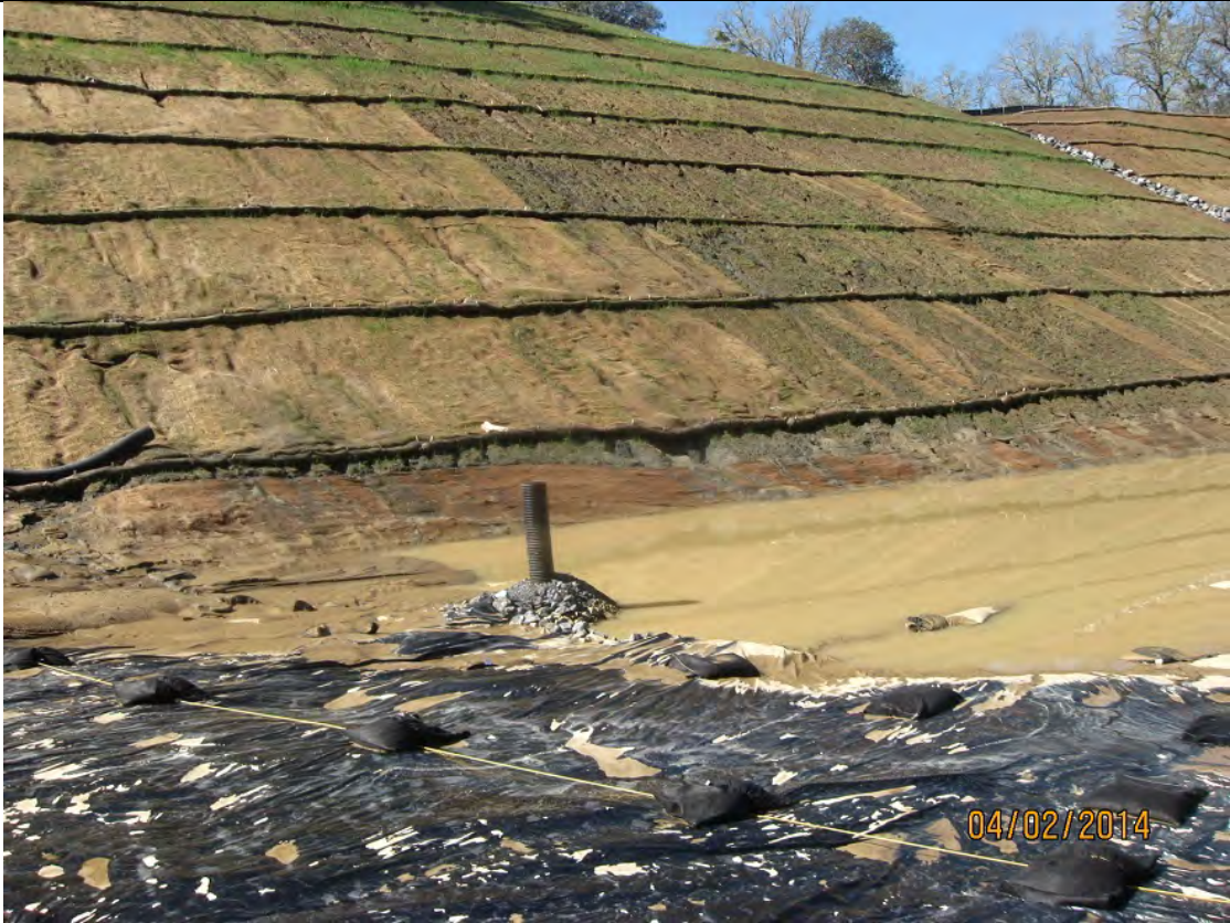
Photo 12: A close-up view of the stormwater basin excavated last year to handle flows from the eroding finished slopes. The basin drains through a perforated drain pipe surrounded by gravel (center of photo).
