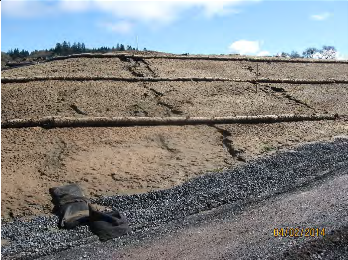
Photo 30: Ineffective erosion and drainage control and gullying on the west side of the U2 line.
