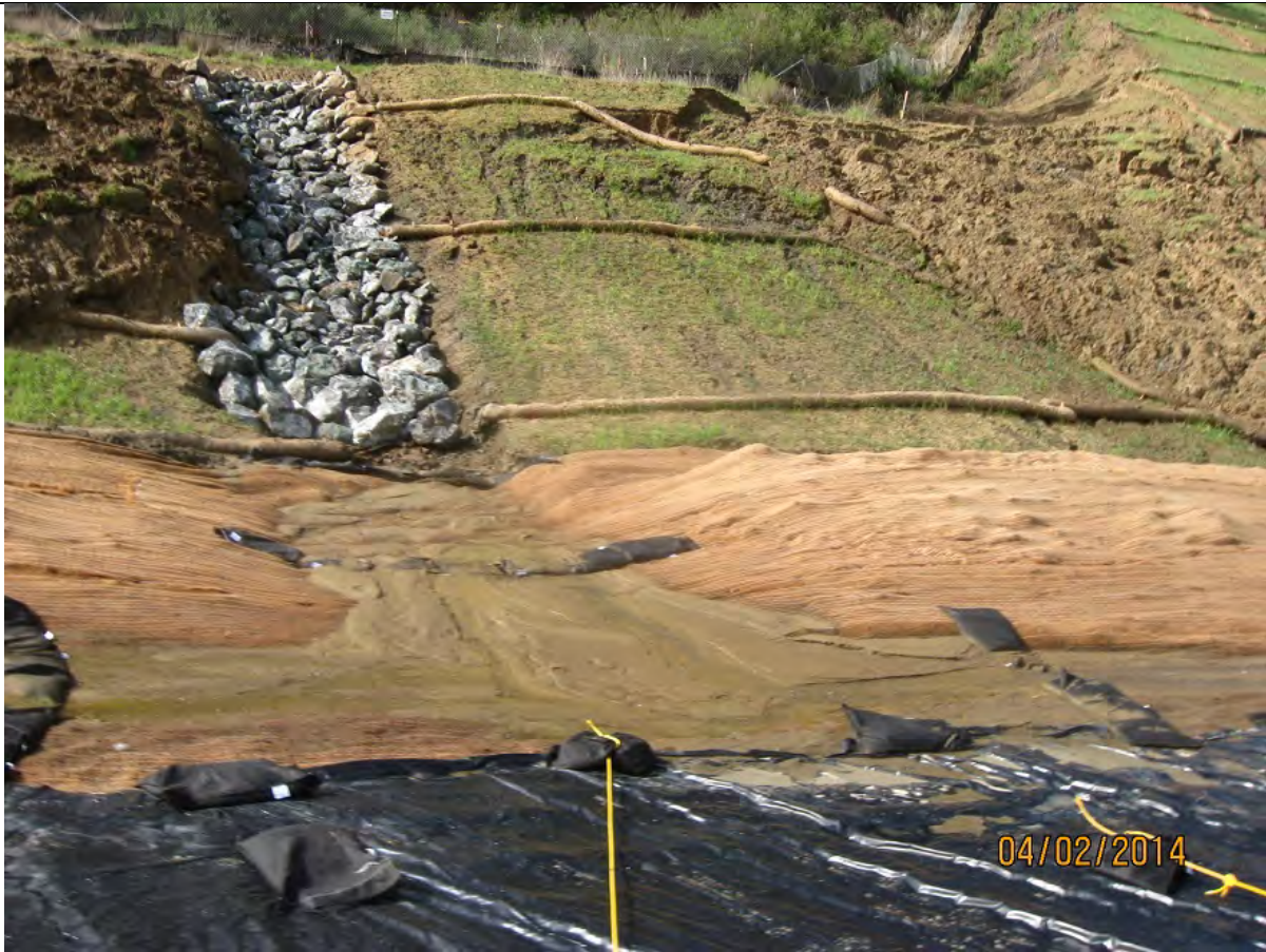
Photo 6: Significant amounts of sediment had been transported from the top of the slope and the failed slope area. This entire area drains to the basin shown in Photo 12.
