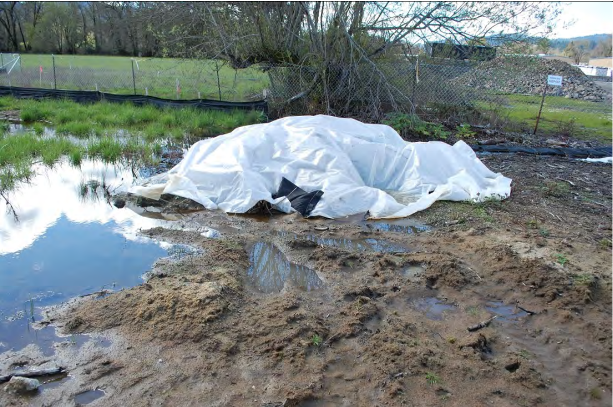
Photo 67: Photo taken looking west at the southern boundary of Spare Time Supply. Vegetation debris is inappropriately stored in standing water and must be relocated.
