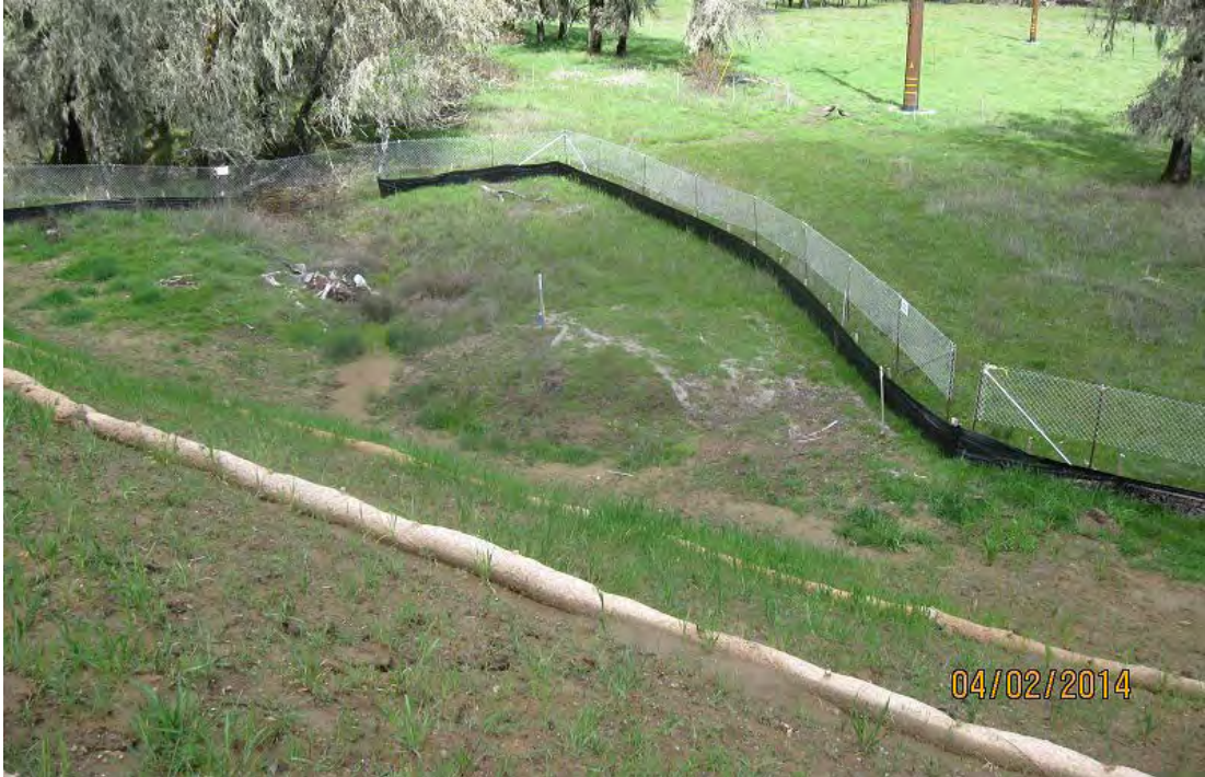
Photo 58: Sediment discharge seen in channel, center left, as a result of eroding embankment (see Photo 59)
