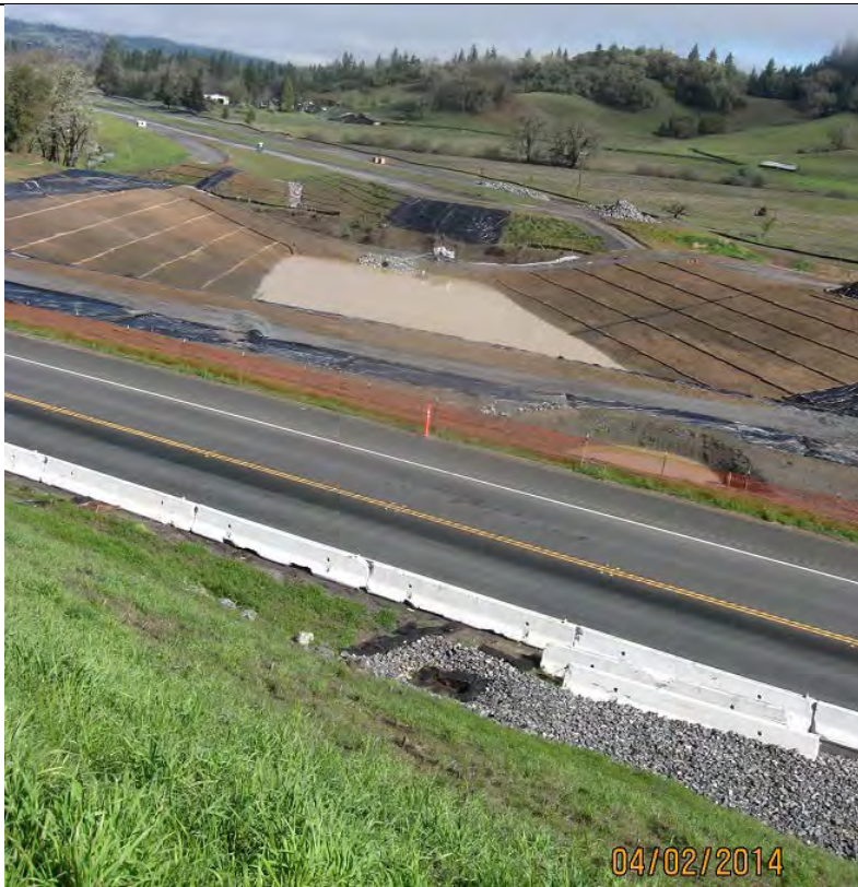
Photo 17: A view of the drain inlet mentioned in Photo 16. A view of the stormwater basin mentioned in Photo 18
