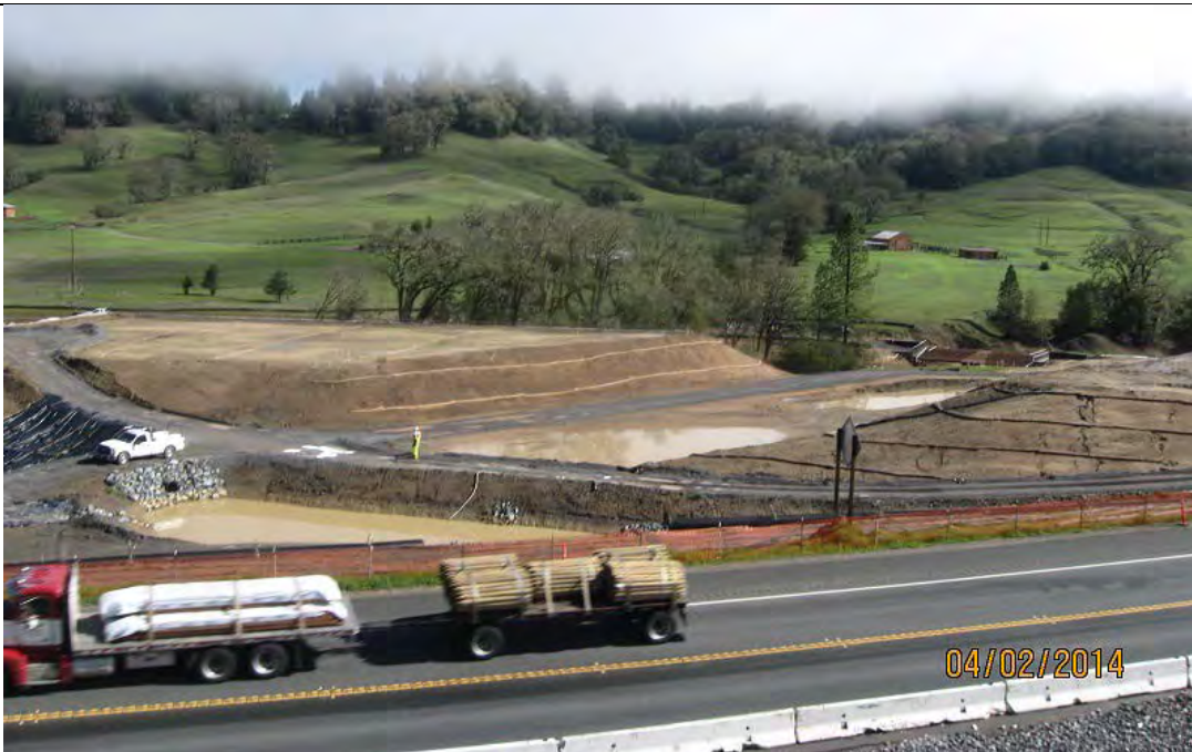
Photo 19: A view across the highway, looking east, at two more areas where stormwater is stored before discharging to South Haehl Creek. The basin in the foreground discharges to Basin 1 and the one in the background discharges to both the basin in Photo 18 and during periods of overflow, directly into South Haehl Creek as described in Photo 54.
