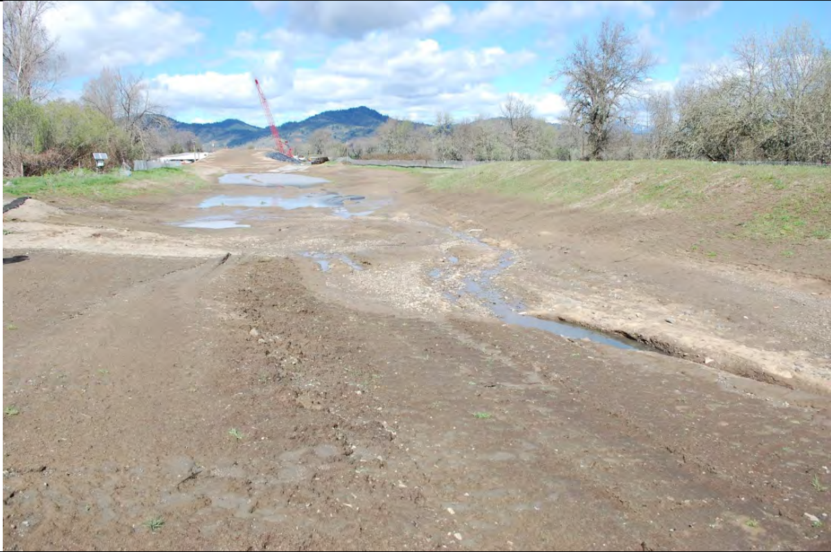
Photo 66: Inadequate erosion control south of Bent 1.
