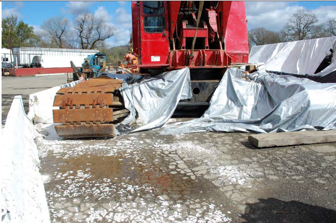
Photo 69: Flatiron's crane had been vandalized twice, resulting in hydraulic fluid spills. Absorbent material was distributed throughout the area. The smell of petroleum product was strong. It had rained the previous two days and the tarps onsite at the time were not large enough to cover the entire spill area.
