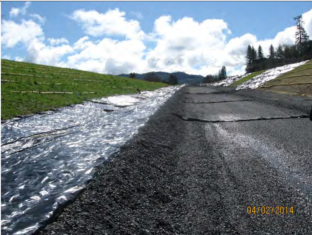
Photo 53: The U2 line downhill from the location shown in Photo 51. Caltrans staff noted that this segment of the gravel road had erosion problems similar to those shown above in Photo 51, but was recently fixed through installation of underdrains.
