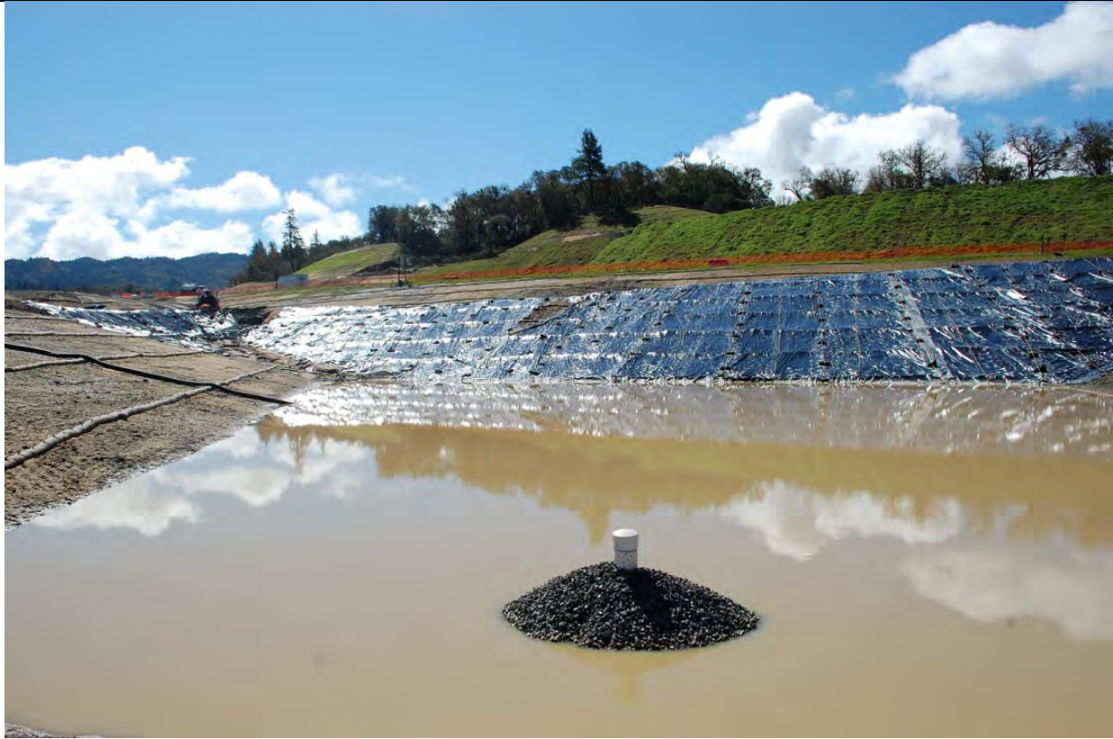
Photo 32: One of two outlets in Basin 1. This is a perforated riser pipe surrounded by gravel for sediment filtration.
