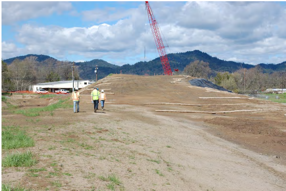
Photo 61: Looking north at Bent 1 at Center Valley Road. The abutment recently had fiber rolls removed and must be replaced.
