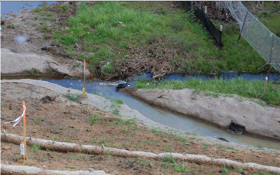
Photo 63: The lower drainage carries storm water from Caltrans disturbed soil areas shown in Photo 62, Photo 64, Photo 65, and Photo 66. It is visibly more turbid than the water from the adjacent drainage that is virtually unaffected by construction operations. Caltrans has been incorrectly representing site discharge by sampling at a location downstream of this confluence. Caltrans must capture representative site samples from a location upstream of this confluence.
