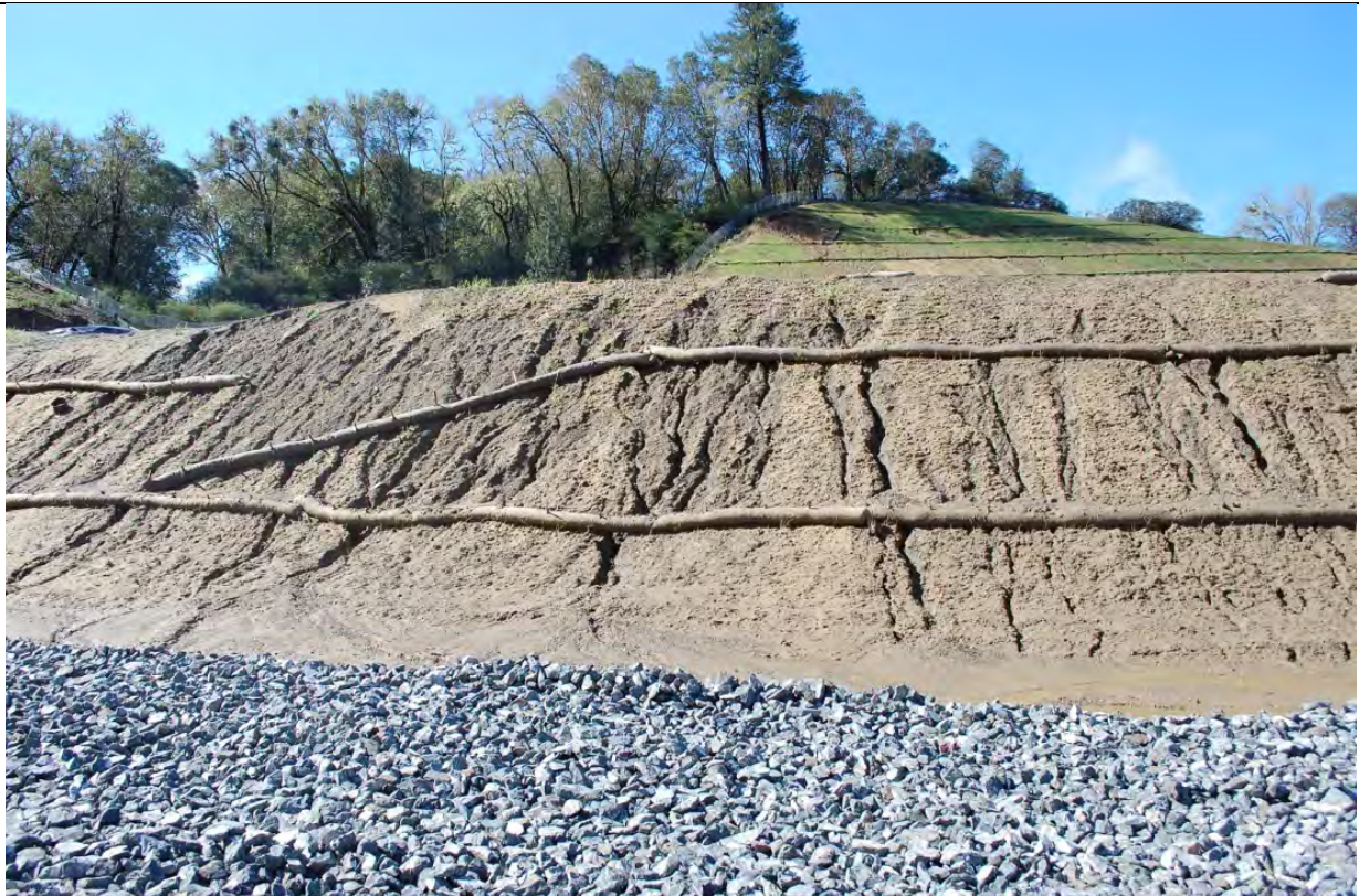
Photo 15: Standing on the shoulder of 101 looking west at the U1 line area. Failure of erosion and sediment control BMPs evident on the temporary slope. The gravel in the foreground was added after the early February 2014 rain event as a sediment control measure. This is part of the same gravel strip as shown in Photo 16.
