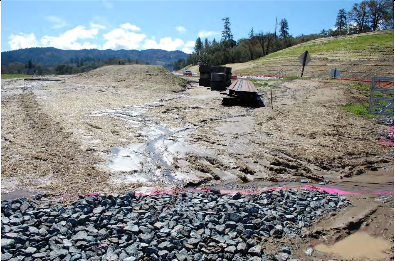
Photo 20: Just southeast of the area shown in Uncontrolled flow is eroding through previously applied straw erosion control. The erosion starts beyond the stockpiled material and adjacent the Highway. This concentrated flow path must be controlled.
