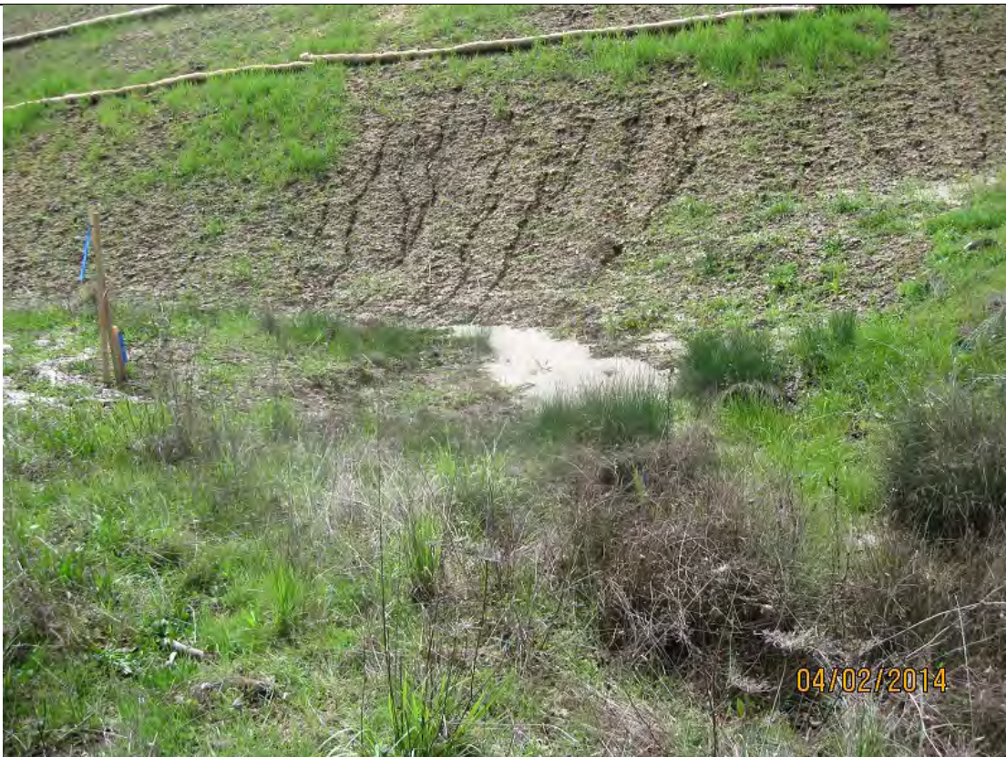
Photo 59: Erosion of embankment discussed above in Photo 58.
