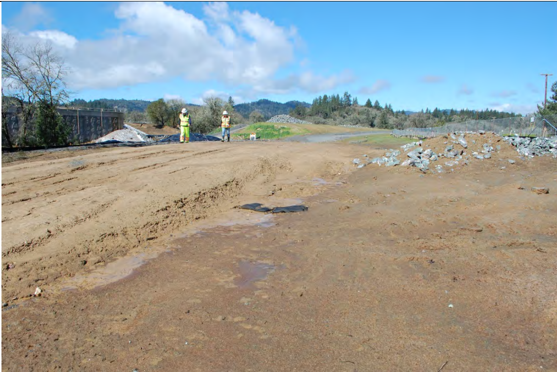
Photo 39: Inadequate erosion and sediment control on and adjacent to the roadway north of South Haehl Creek, looking north on the “U4” line.
