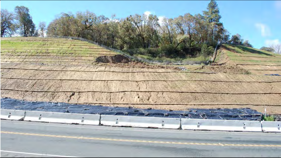
Photo 2: Final grade slope in “U1” area, west of 101, South Haehl Creek watershed. A large portion of the slope failed in an area that exhibits evidence of pre-project slope failure. According to Caltrans staff, this failure had started 2-3 weeks before the inspection. Caltrans staff also mentioned that their geotechnical engineers were working on a solution.
