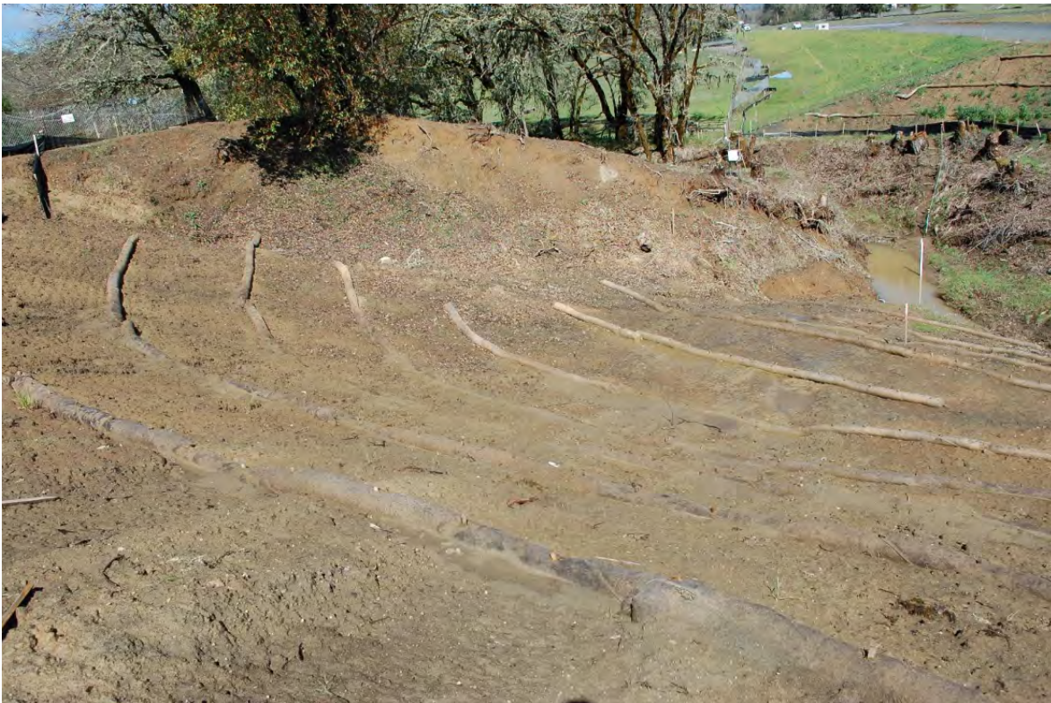
Photo 36: Standing at the top of Basin 1, looking at the south bank of South Haehl Creek. The top rows of fiber rolls were inundated with sediment.
