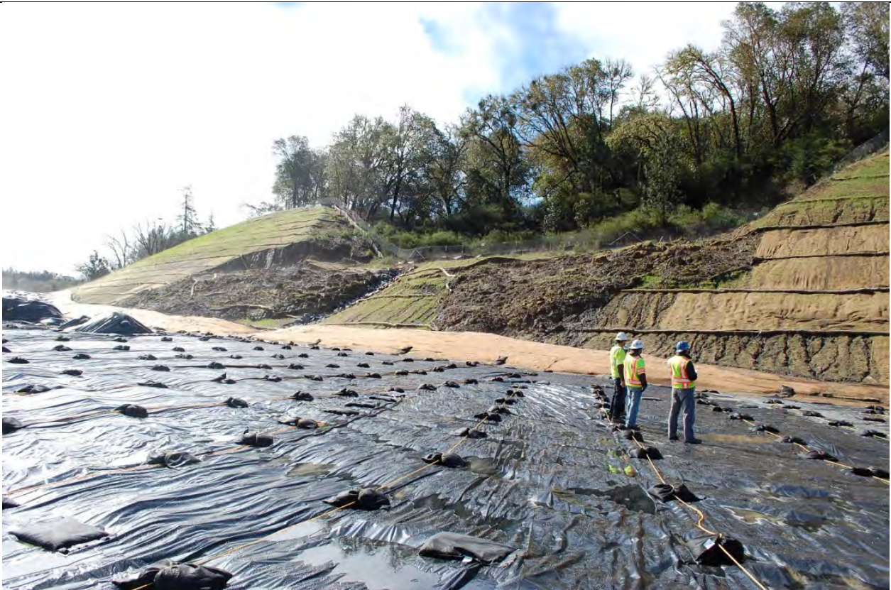
Photo 8: View of slope failure across a large area covered with plastic as a temporary erosion control fix.
