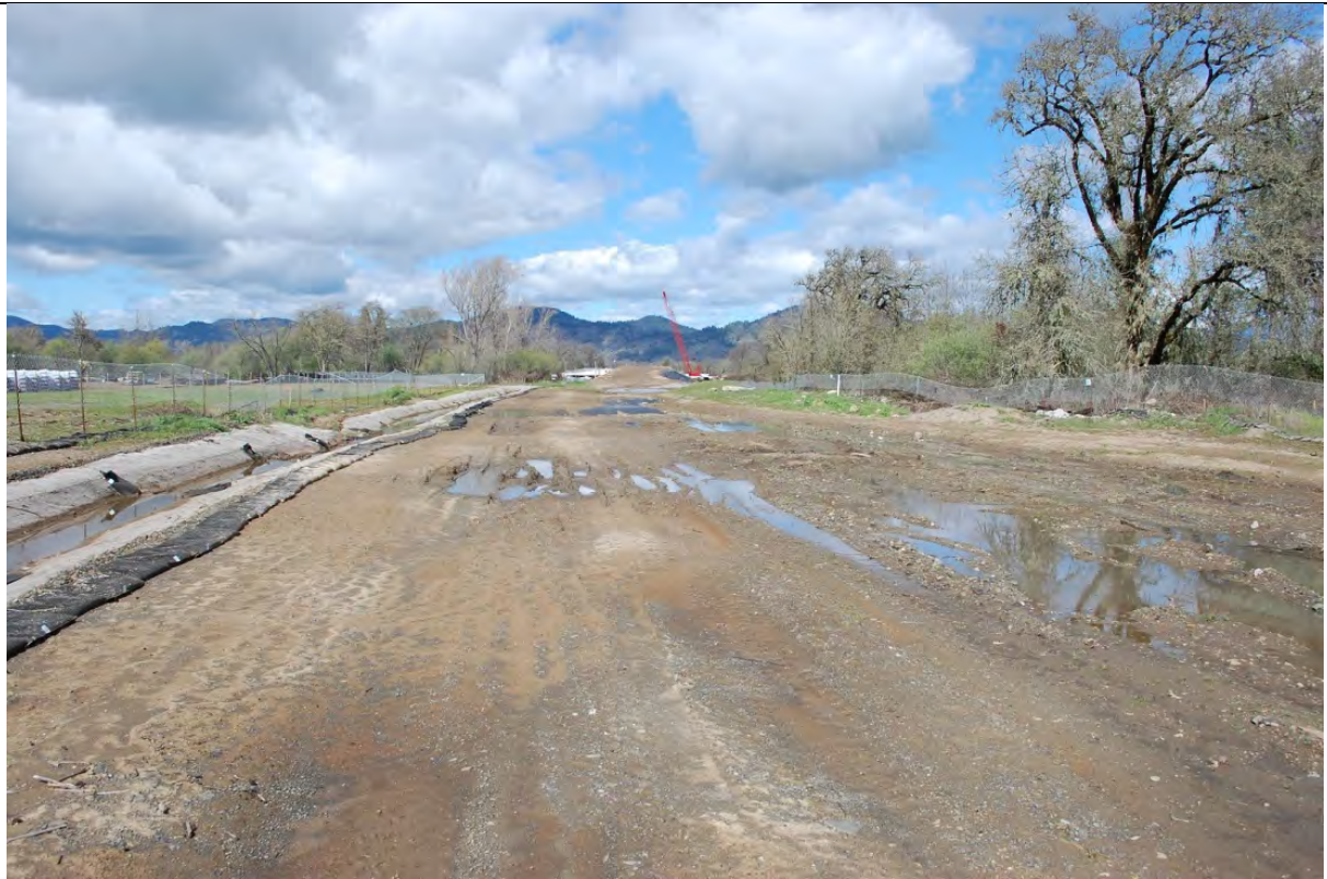
Photo 65: Inadequate erosion control south of Bent 1.
