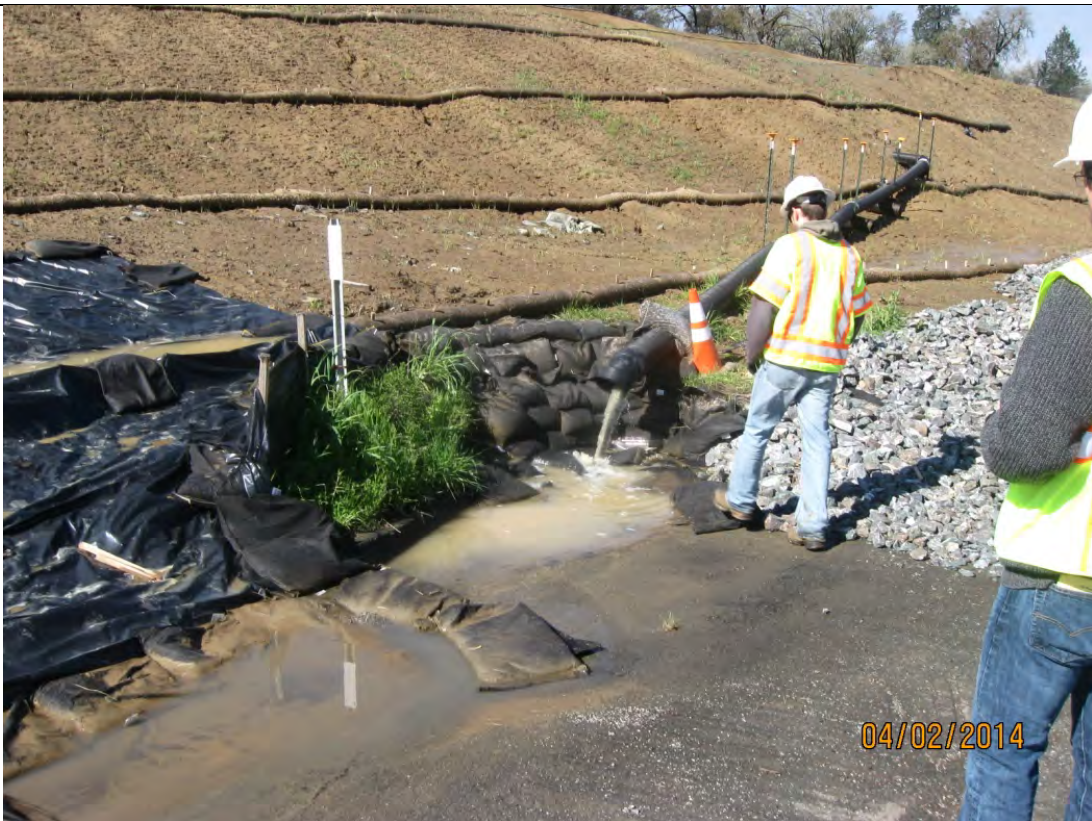
Photo 13: The basin shown in Photo 12 discharges to this drainage inlet on Hwy 101 before being carried under the highway to the basin shown in Photo 21.
