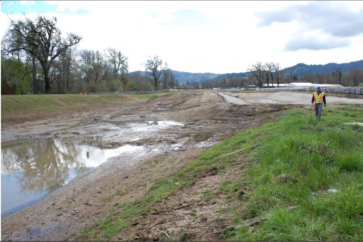
Photo 64: Inadequate erosion control south of Bent 1.
