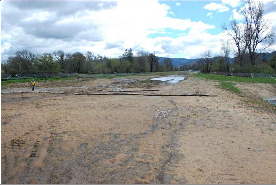
Photo 62: Looking south at disturbed area south of Bent 1. This large area has generally inadequate erosion and sediment controls. This area discharges to a tributary of Baechtel Creek at the location shown in Photo 63.
