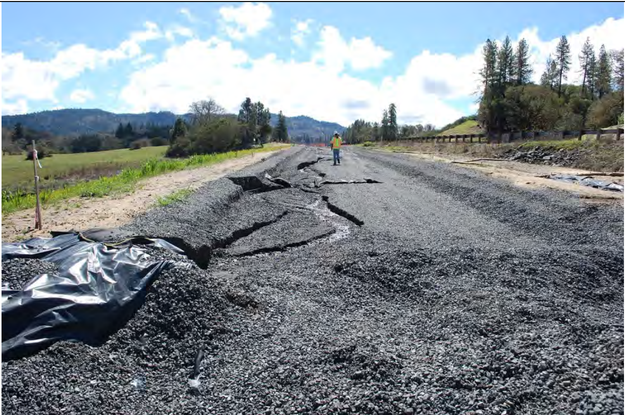
Photo 51: Looking north at the U2 line, south and upgradient of the area shown in Photo 50. The gravel road was significantly incised and sediment had been transported downstream to South Haehl Creek. The inlet is beneath the black plastic, shown in the lower left of the photo (see Photo 52).
