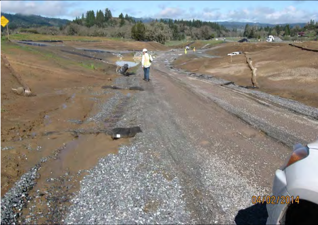
Photo 26: Looking north on the U2 line toward the basin shown in Photo 27 and Photo 28. Sediment had inundated this check dam during the previous rain event and gulying occurred downstream as a result.
