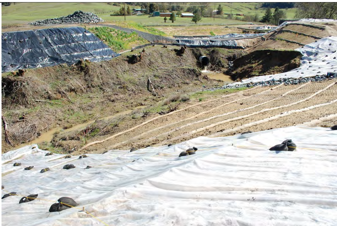
Photo 37: Standing at the top of Basin 1, looking at the south bank of South Haehl Creek. The area in the foreground with plastic sheeting is just upstream of the area shown in the previous photo. All plastic was recently placed to cover the eroding bank.
