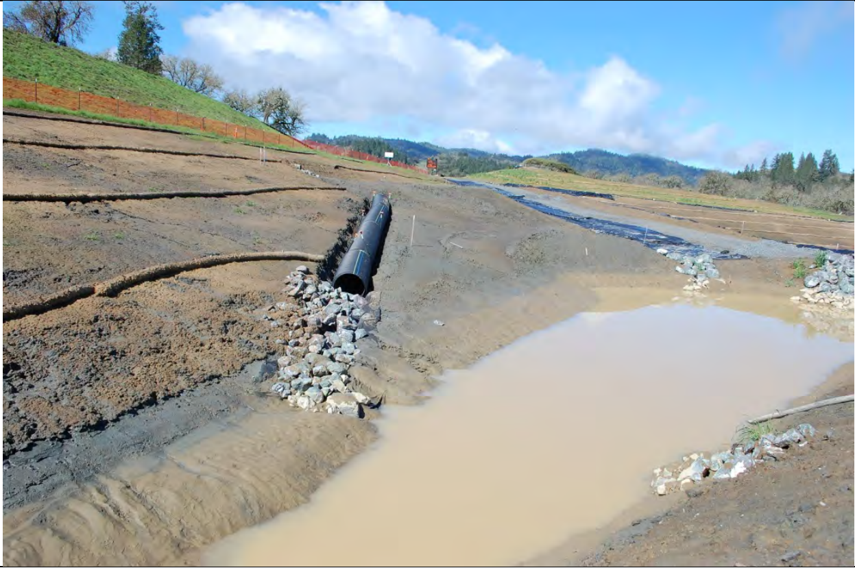
Photo 28: This basin receives flow from the disturbed area west of Hwy 101, the basin in Photo 21 and discharges to Basin 1.
