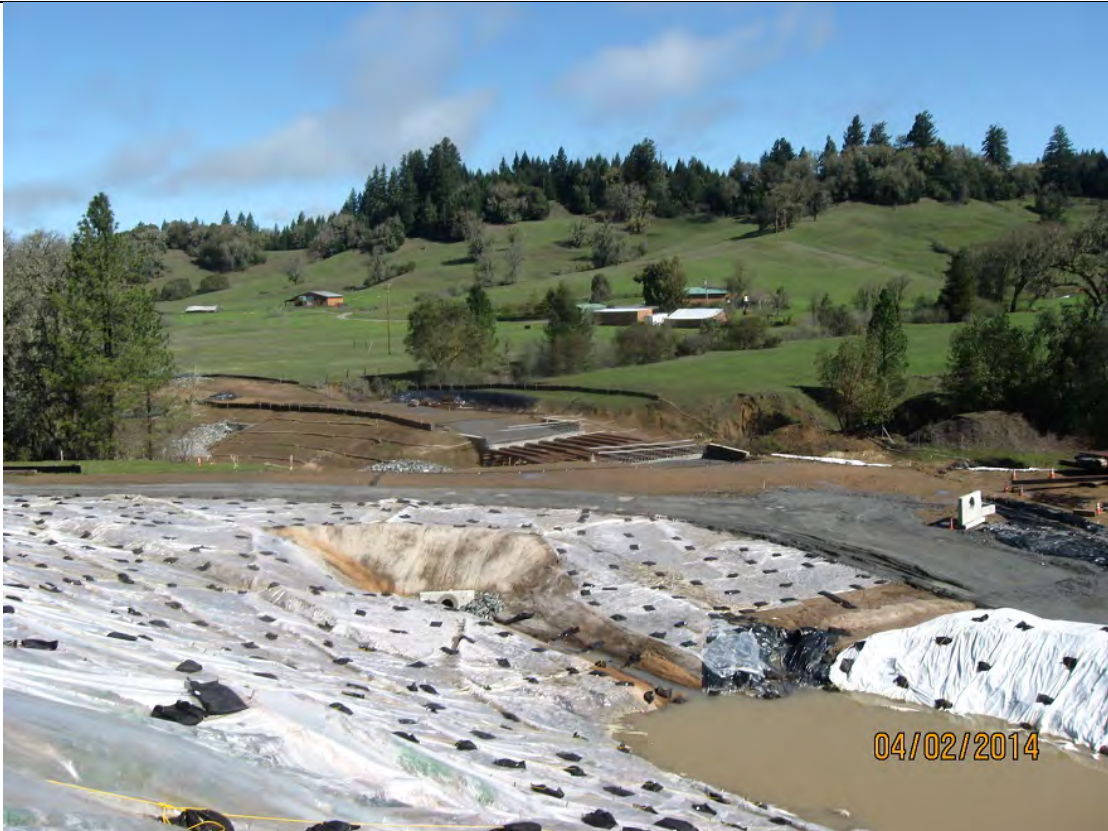
Photo 25: A view of the storm water basin on the east side of the “U2” line. This basin discharges directly to South Haehl Creek and receives storm water runoff from the east side of the future northbound Haehl interchange off-ramp.
