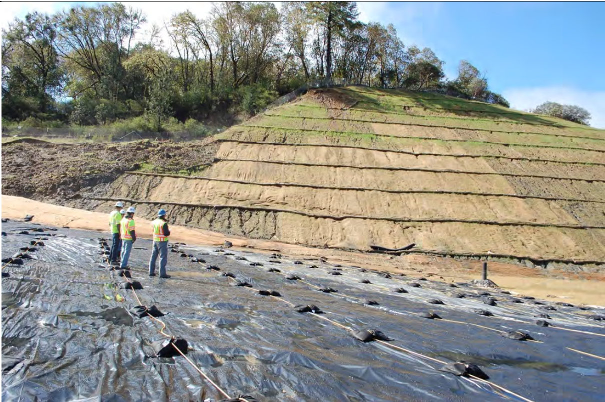
Photo 9: Finished slope just north of the slope failure. This is one of the few slope locations with rolled erosion control fabric. The fabric was placed sometime after the early February 2014 rain event. A new slope failure is starting at the top left of the slope where the tree shadow is. The ad hoc storm water basin is visible right center.
