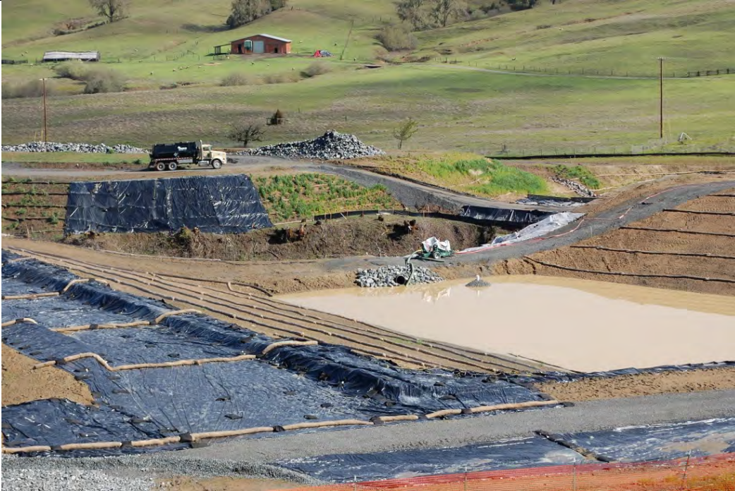
Photo 18: A view across the highway, looking east, at the largest stormwater basin (hereinafter "Basin 1." Water discharges directly from this basin into South Haehl Creek. Caltrans has been using water trucks, like the one seen in the distance, to pump and truck turbid water from this and other basins to the Willits Wastewater Treatment Facility. Contractor staff said that three, 5,000 gallon water trucks were being operated throughout the day (and 4 the previous day) and could transport approximately one load per hour.
