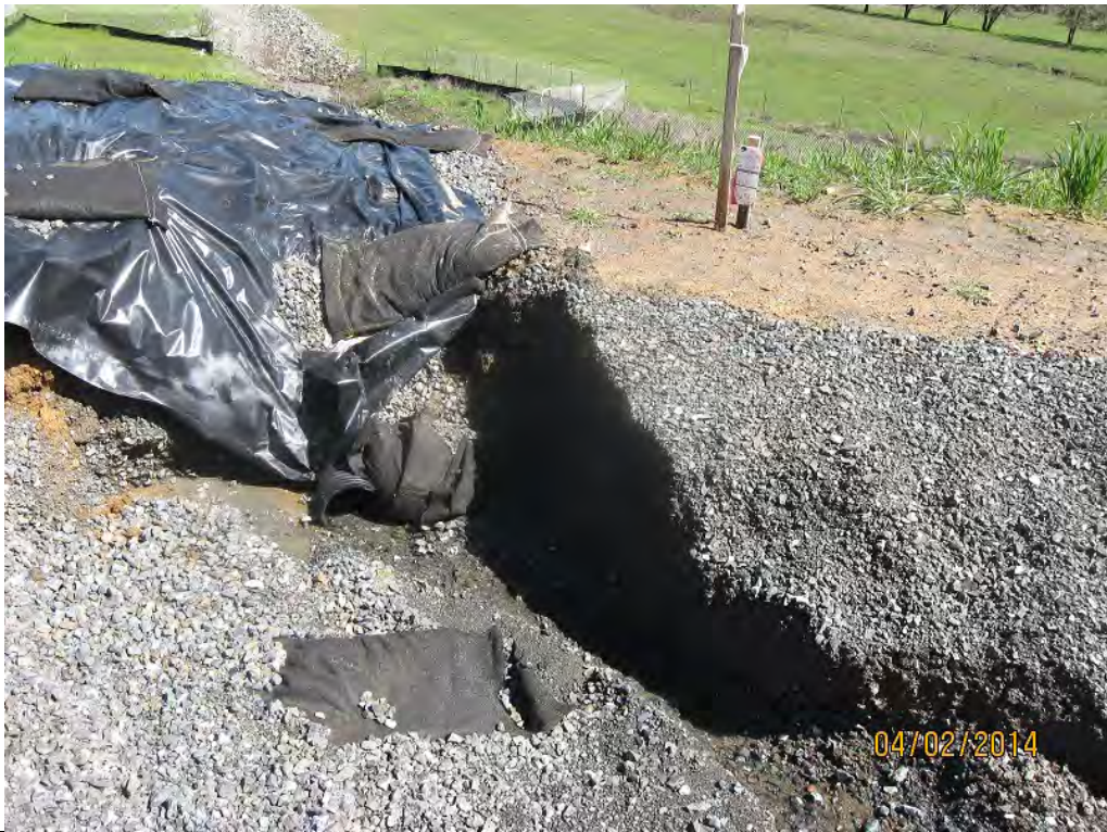
Photo 52: A view of the inlet shown in Photo 51.
