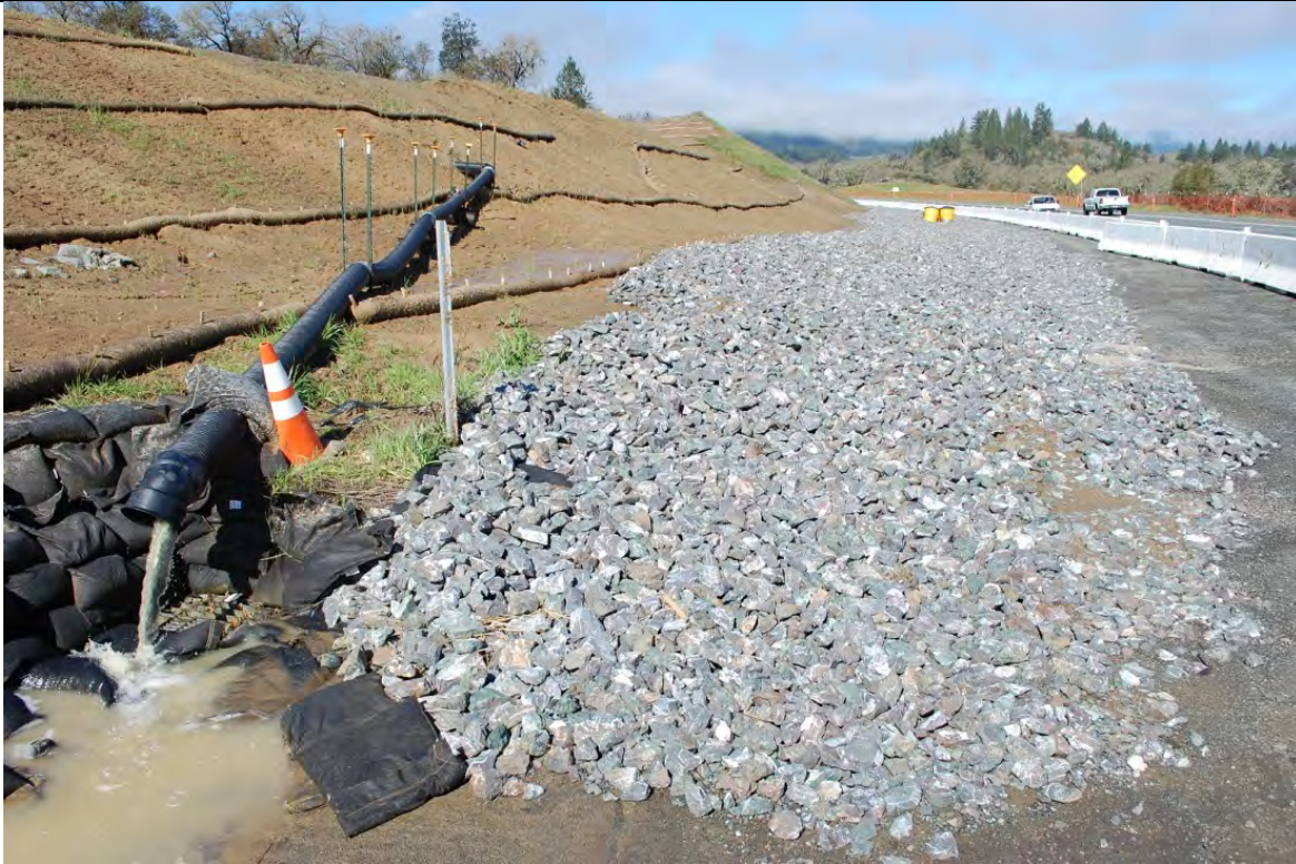
Photo 16: Looking north along the shoulder of Hwy 101 where gravel was placed as a sediment control. The road slopes downward and the gravel extends to the location of a drain inlet (see Photo 17) that transports stormwater under the freeway to the basin shown in Photo 28.
