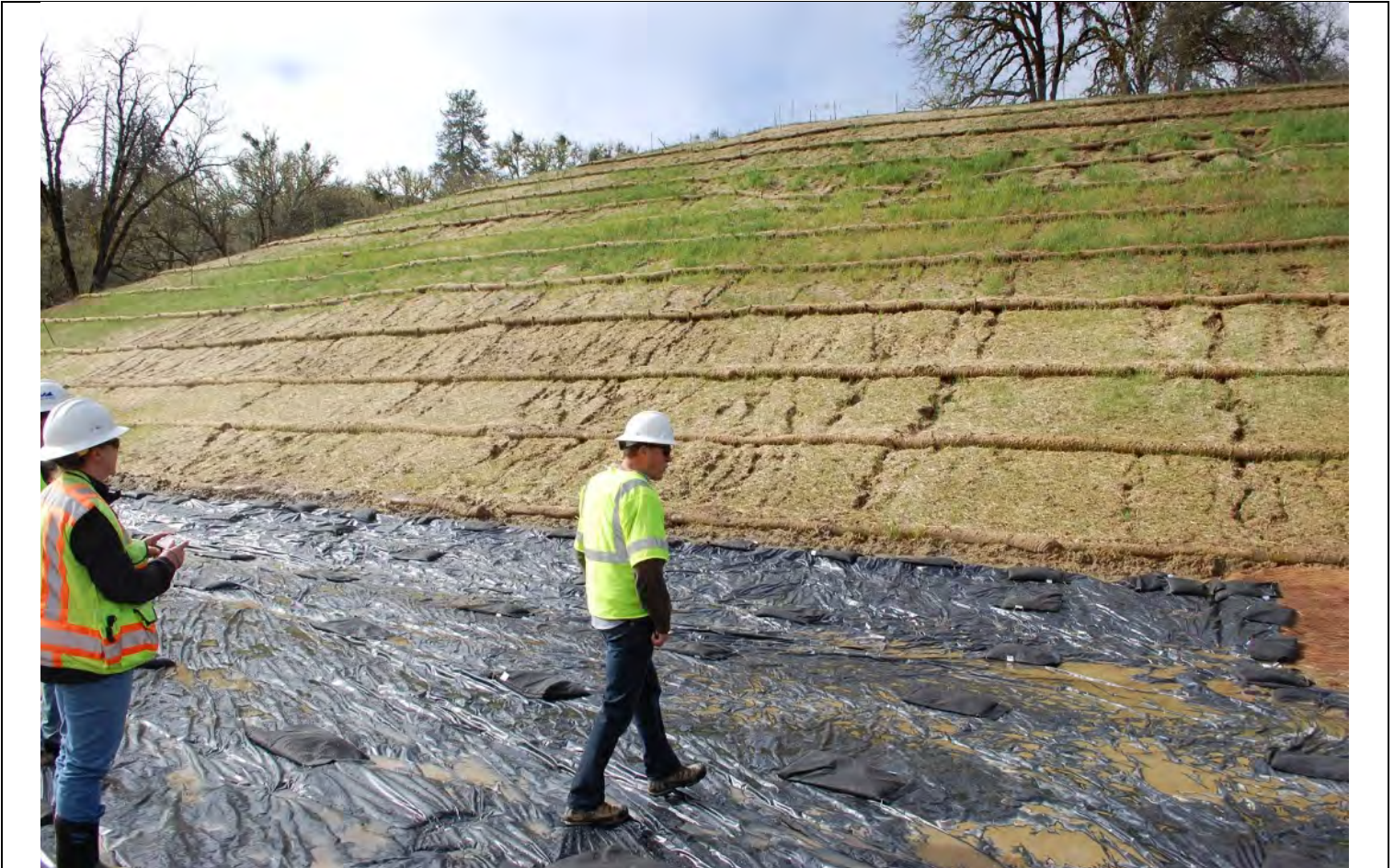
Photo 1: Final grade slope in "U1" area, west of 101, South Haehl Creek watershed. Rilling was evident. Fiber rolls and bonded fiber matrix with seed had been applied last year. Caltrans and contractor staff noted that the slopes could only be repaired by regrading, which has not been done due to the saturated soil conditions and lack of access.
