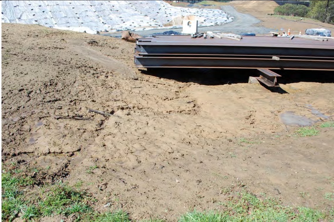
Photo 46: Looking west at a material storage area, just south of South Haehl Creek at the bridge 0129 abutment. Inadequate erosion and sediment controls.
