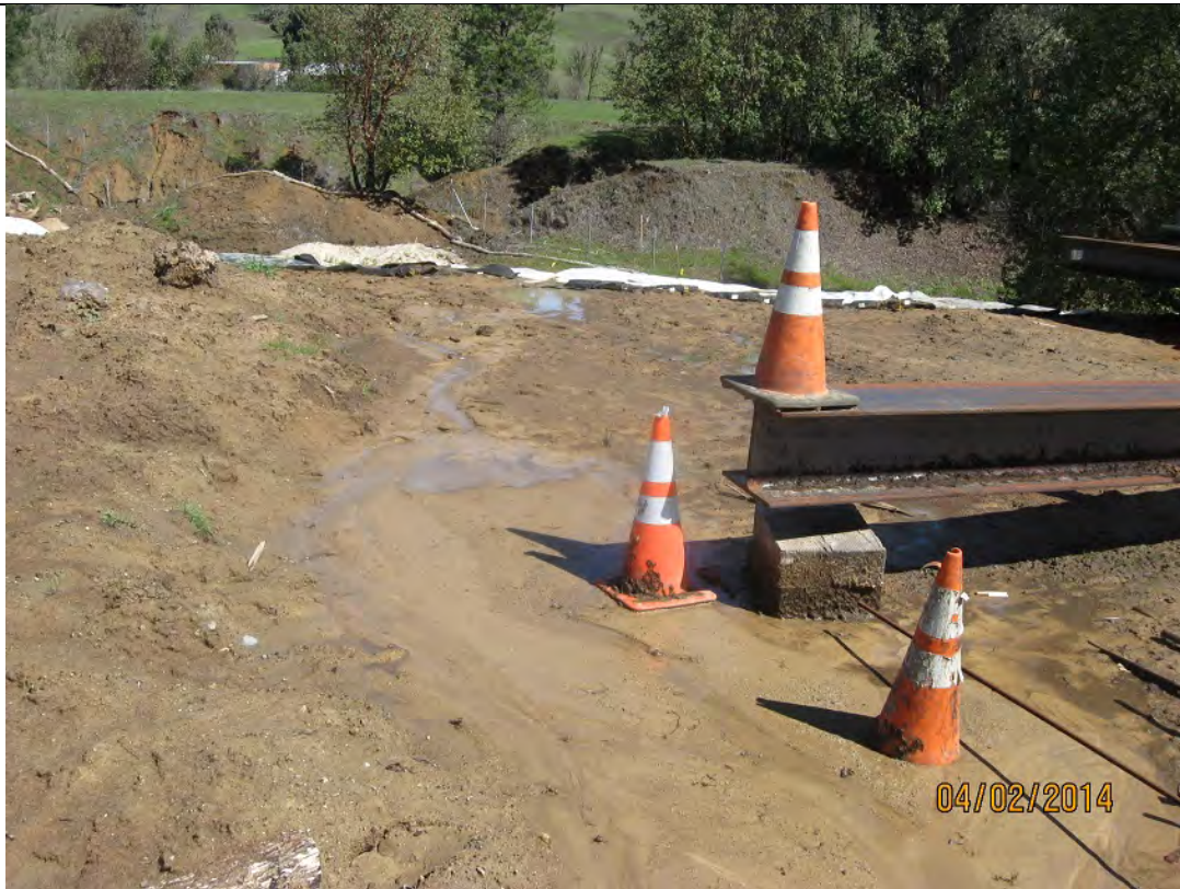
Photo 47: Looking east at a material storage area, just south of South Haehl Creek at the bridge 0129 abutment. Inadequate erosion and sediment controls. The concentrated flow path runs toward south Haehl Creek.
