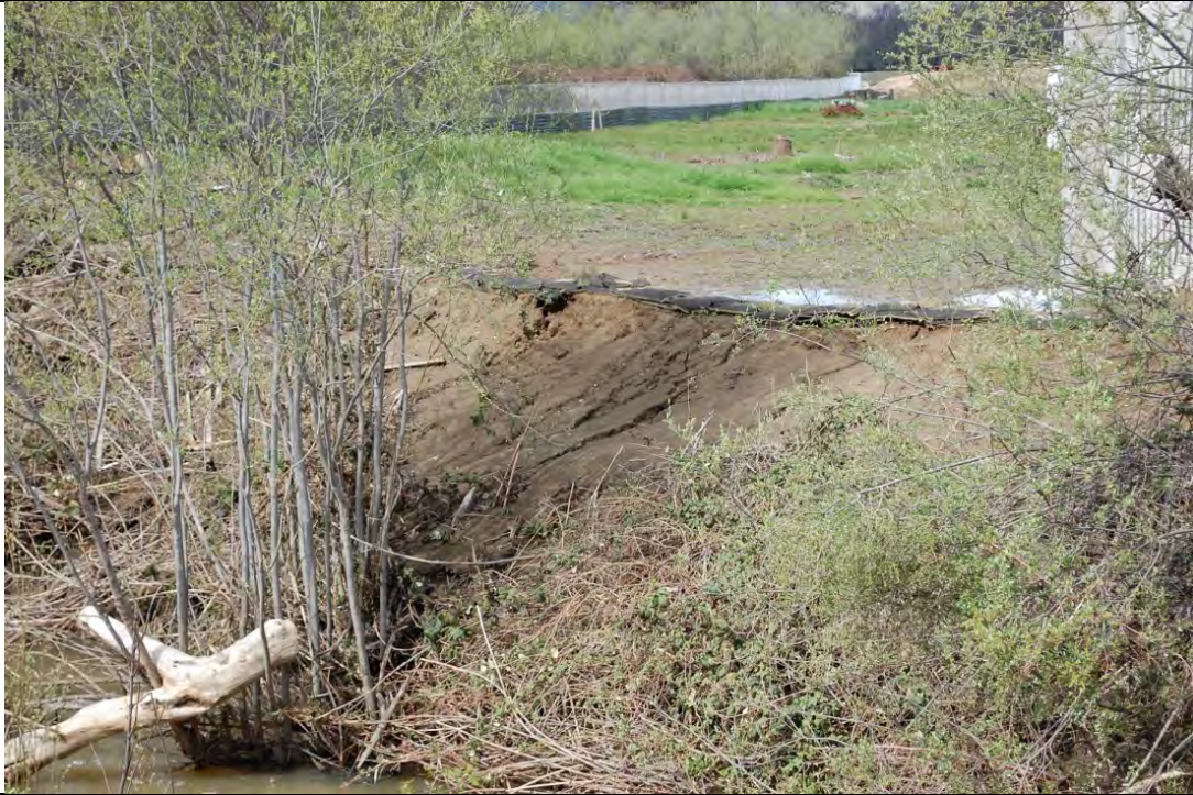
Photo 72: Looking northwest. Sediment discharge to Baechtel Creek at Pier 4 as a result of inadequate erosion control and failed sediment control. Erosion and sediment control must be provided.
