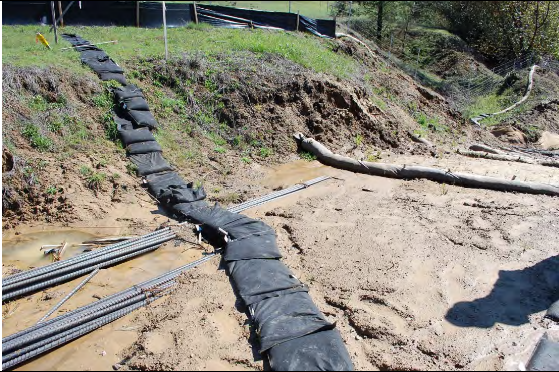
Photo 44: Looking south toward South Haehl Creek, just south of Drainage System 24. The rebar was not moved, according to staff, because it was too heavy to move without heavy equipment.
