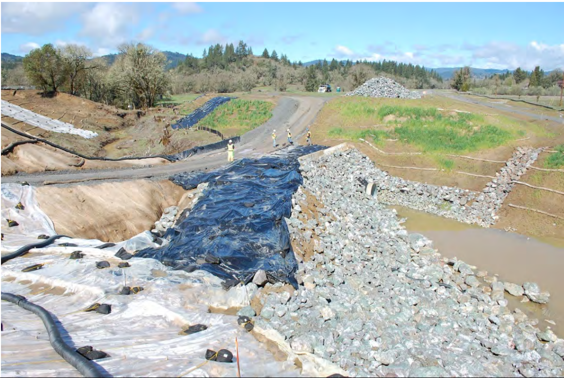
Photo 38: Standing just east of the previous photo, looking north at the temporary culvert for South Haehl Creek. The rock was placed after the early February 2014 rain event to protect the eroding the creek banks.
