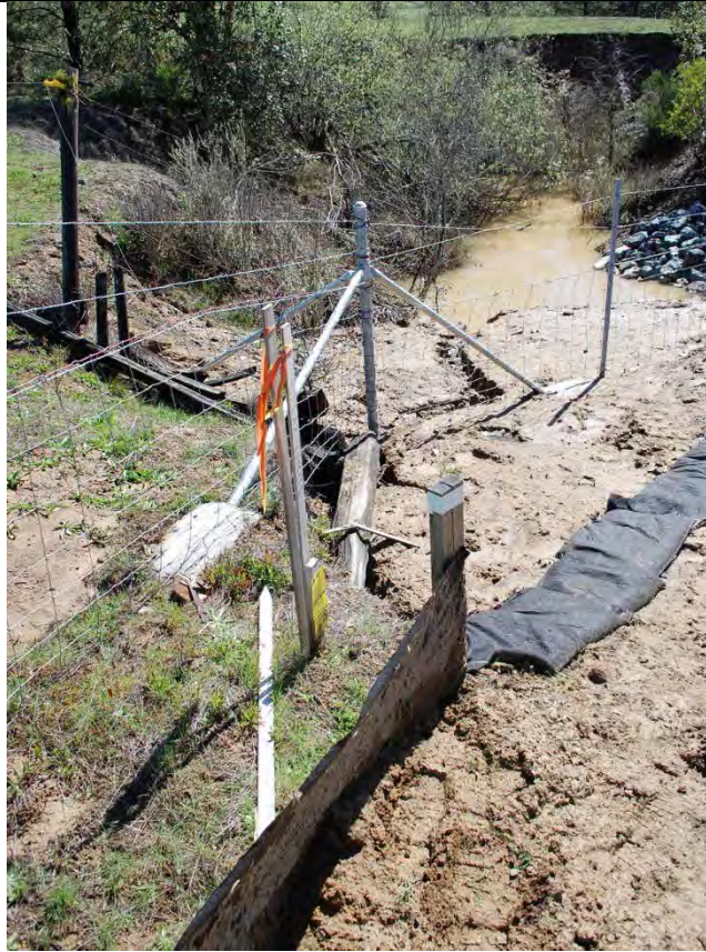
Photo 42: Looking southeast at Drainage System 24 before it enters a culvert and discharges to South Haehl Creek. A large gully has formed developed into the channel, as seen in the center of the photo. The steel fence is the Caltrans right-of-way fence. Caltrans staff said they were limited to fixes within their right-of-way, however, the disturbance on the other side of the fence was created by Caltrans and is Caltrans's responsibility to stabilize.
