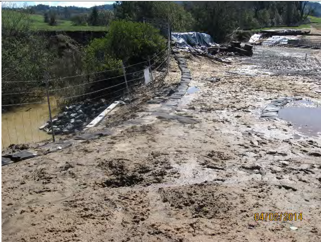
Photo 41: Looking south at Drainage System 24 before it enters a culvert and discharges to South Haehl Creek. There was inadequate erosion and sediment control in this area. This area must be stabilized.
