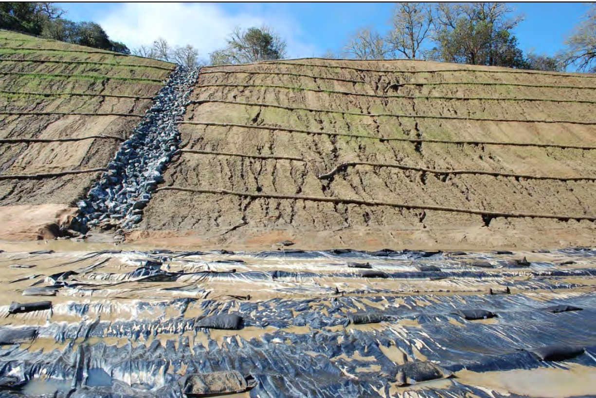
Photo 11: A view of the gullied, finished slope with rock-lined drainage ditch, above the storm water basin. The temporary plastic was covered with muddy water, likely residual from higher basin levels. Note failing fiber rolls. Before the plastic had been placed, sediment was removed from the basin and spread over the surrounding area to provide greater basin storage volume.
