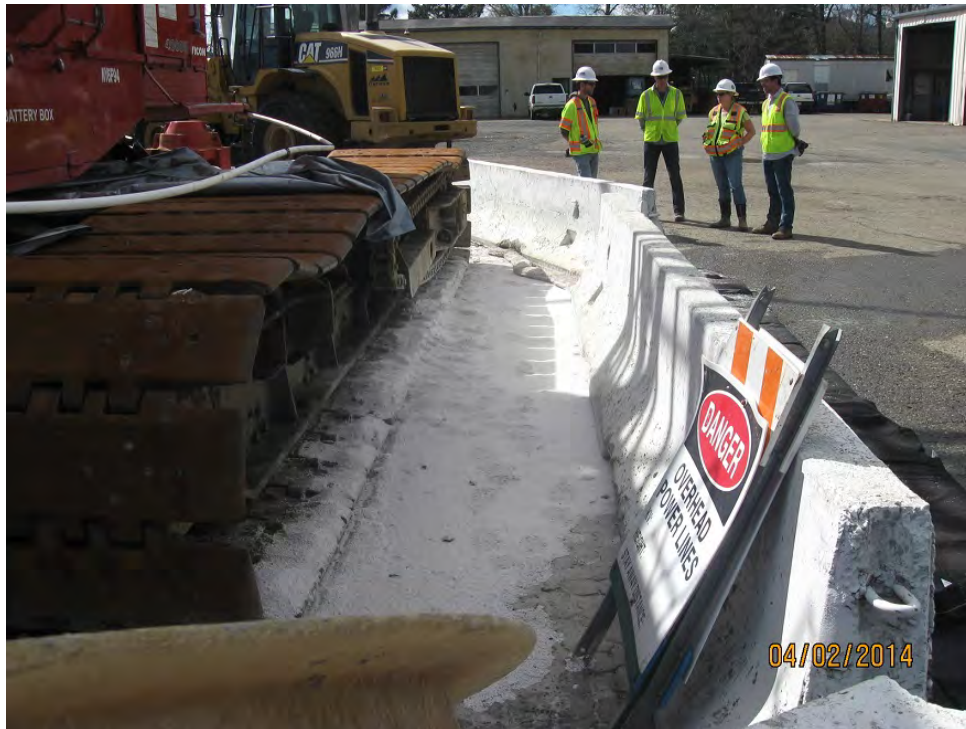
Photo 70: Absorbent material had been applied to absorb hydraulic fluid. Gravel bags along the perimeter appeared to have absorbed fluid. Caltrans must provide the Regional Water Board with information detailing the dates the hydraulic lines were cut as well as documentation of appropriate clean-up and disposal activities.
