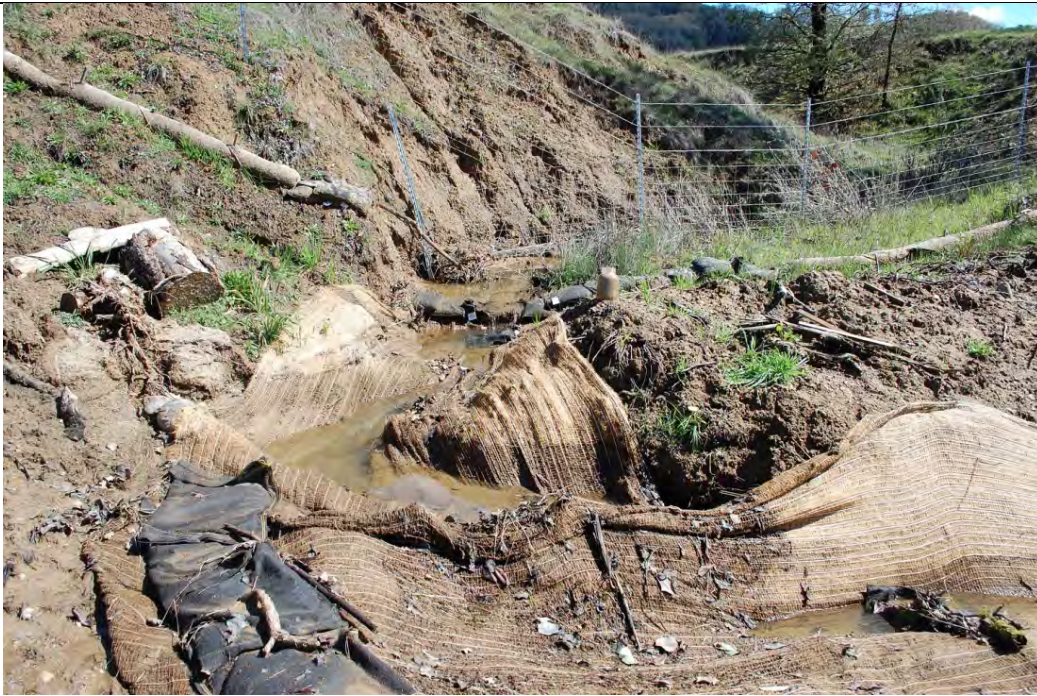
Photo 45: A closer view of the area shown in Photo 44, upper right. This watercourse runs into Caltrans's project limits from the Schmidbauer property, just before discharging to South Haehl Creek. Because a stable drainage path to South Haehl Creek was not planned for and provided, drainage has eroded the creek bank and transported sediment to South Haehl Creek. A stable drainage path must be provided. Plans for the final drainage configuration must be approved by the Regional Water Board. Biotechnical elements should be incorporated as appropriate.
