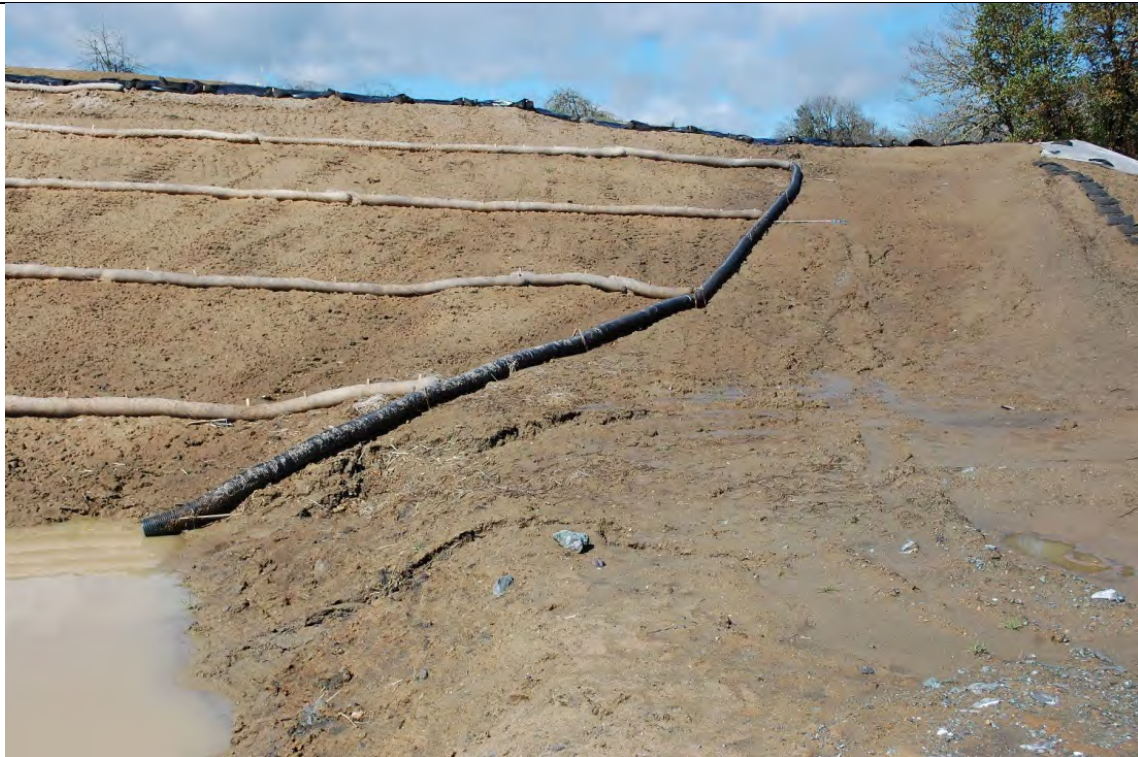
Photo 34: At the northern end of Basin 1, looking west. This dirt area was unstabilized and eroding. This area must be stabilized.
