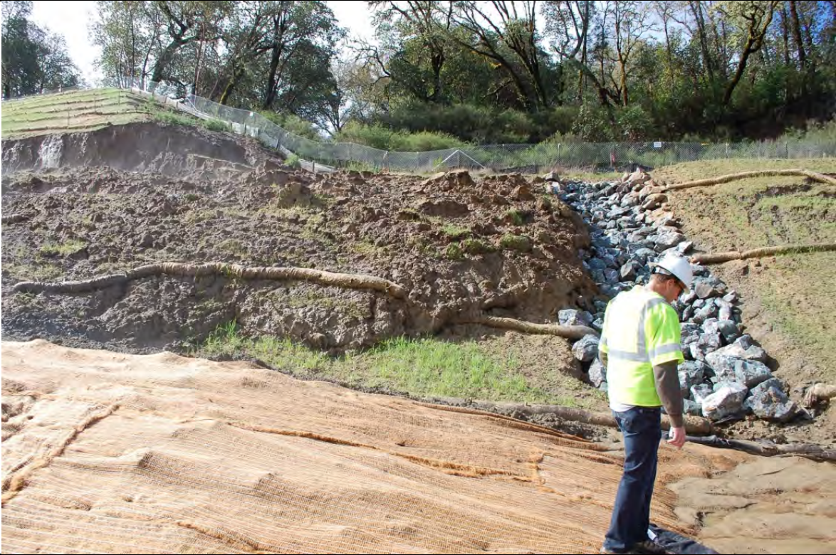
Photo 4: A close up of the slope failure shown in Photo 2. A rock-lined drainage ditch had been constructed to carry stormwater from the top of slope. Photo 5 shows disturbed conditions at the top of the slope.
