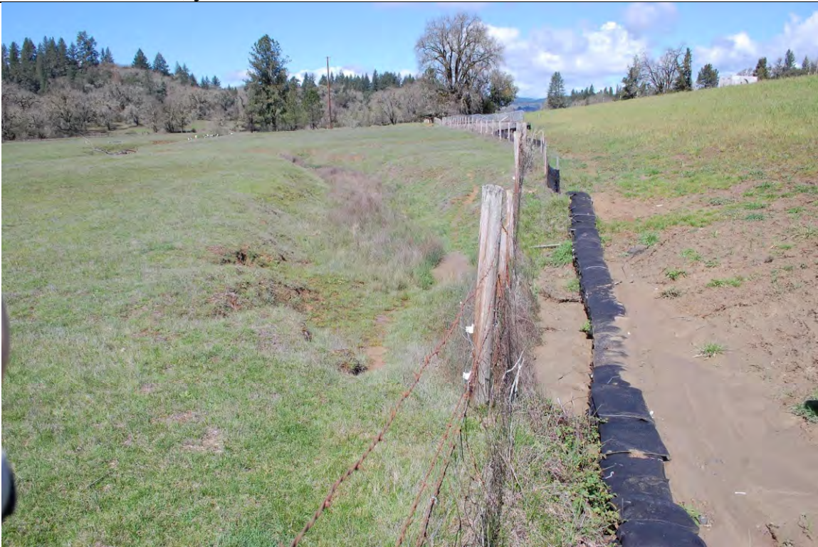
Photo 57: Looking north. Erosion and sediment transport and discharge off-site at the toe of slope along the U3 line. The contractor’s Water Pollution Control Manager discussed plans to remove sediment and install erosion control fabric and gravel bag check dams within the channel. I do not know exactly where this off-site drainage discharges.
