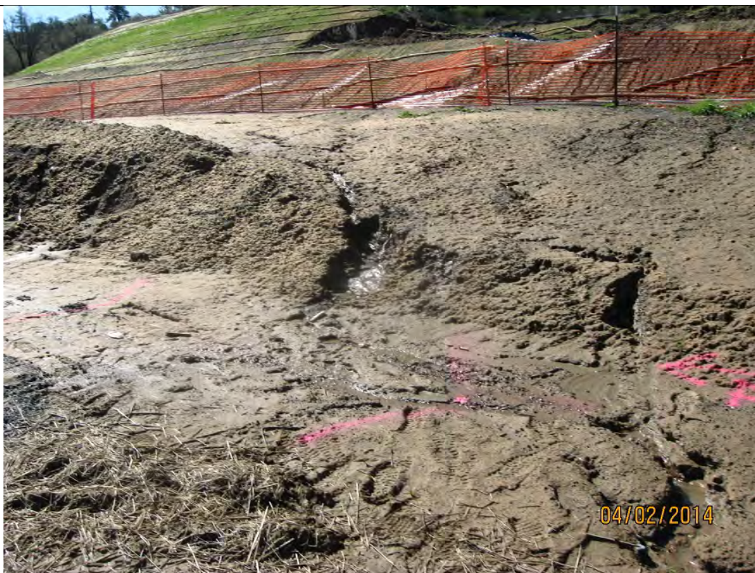
Photo 23: Just north of the basin shown in Photo 21. Erosion from uncontrolled run-on.
