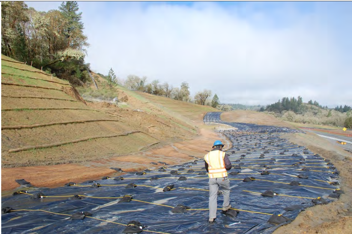
Photo 3: Looking north. The inactive roadway in the U1 area had been covered with plastic and gravel bags for erosion control. The plastic had been placed just before the previous rain event. The Flatiron representative said that placement of plastic resulted in an NTU decrease of “thousands” at the discharge point shown in Photo 13. The slopes to the left were finished to final grade last year, whereas the slopes on the right are still scheduled to be excavated. The slope failure shown in Photo 2 is on the middle-left of this photo.
