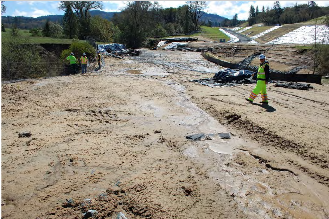
Photo 40: Looking south toward South Haehl Creek, standing at approximately the same position used in Photo 39. Inadequate erosion and sediment control.
