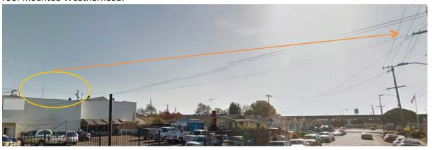
The Boost Mobile front side connection shows a clearly undersized PG&E drop when compared to the building services wires emerging from the weatherhead.
