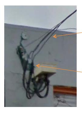
Boost Mobile - Building service wires. 2x 4/0 copper wires per phase. Capacity of 400Amps within the building The Line drop from Derby Street is similarly small.
