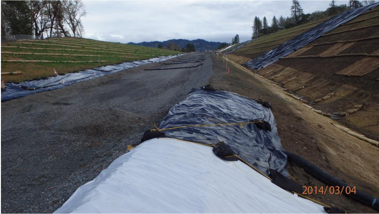
Corrective Action Photo 5C: Looking south along the U2-Line
