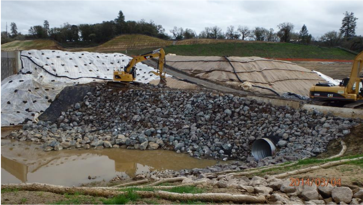
Corrective Action Photo 1E: Crew installing ¼ ton RipRap slope stabilization along eastern bank of the culvert crossing. Looking southwest at the culvert crossing and Bridge Number 10-0129 RL
