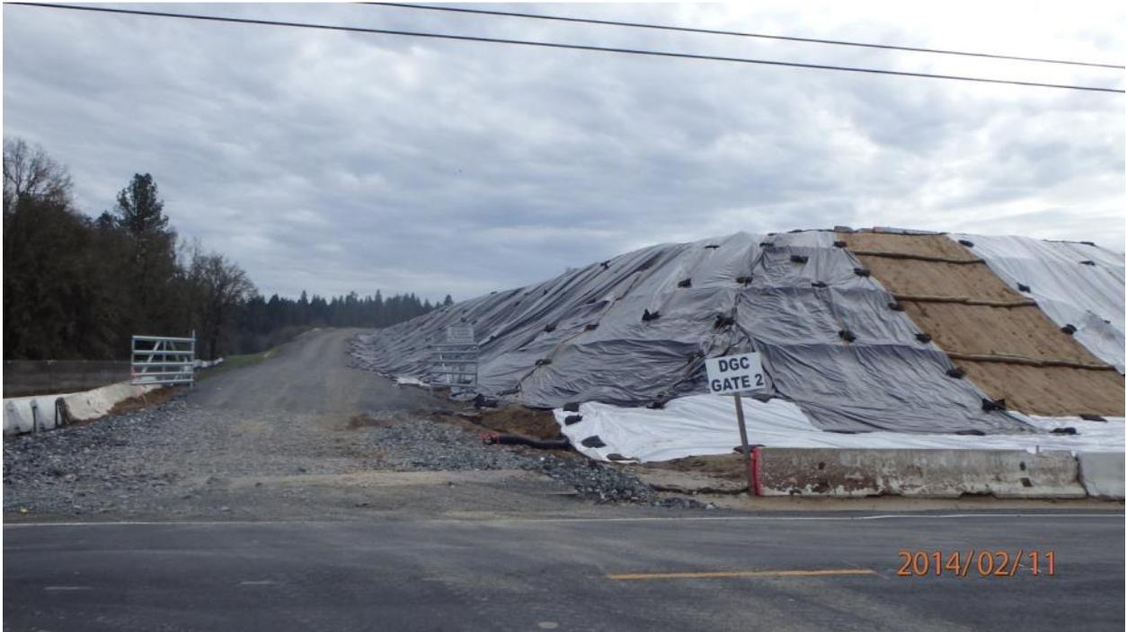
Additional Corrective Action Photo 1: Plastic cover at Bridge 10-0157 Abutment 1
