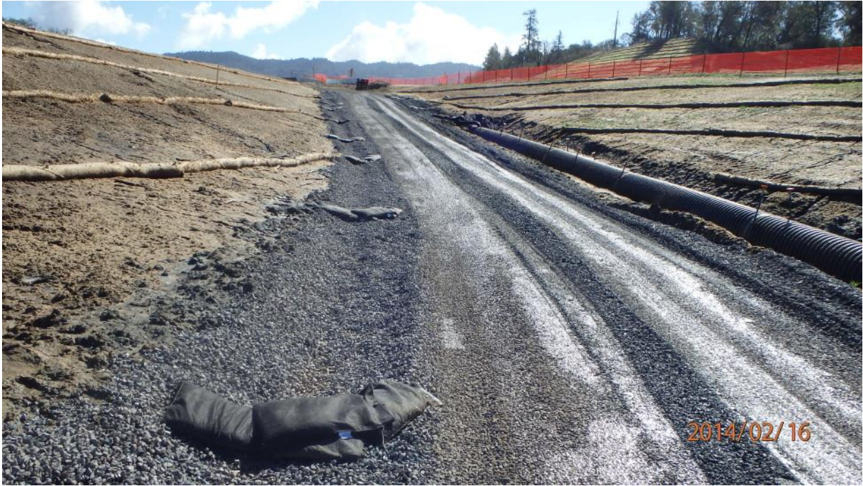
Corrective Action Photo 2B: Stabilized ditches along the winter access road at the South Haehl Creek Interchange
