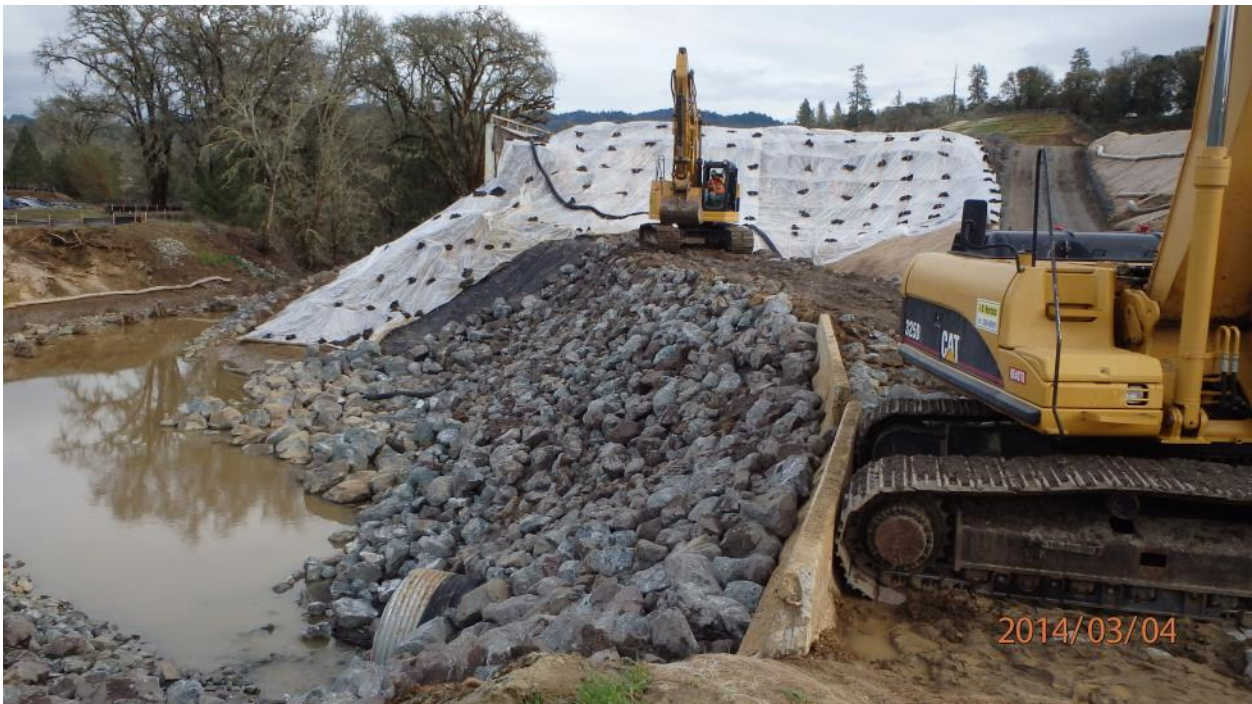
Corrective Action Photo 1F: Looking south at the culvert crossing and Bridge Number 10-0129 RL
