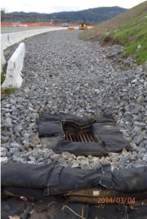
Corrective Action Photo 6A: Drainage inlet has been stabilized with 3-6" drain rock, filter fabric and gravel bags. Looking south along Highway 101 at the base of the U1-Line
