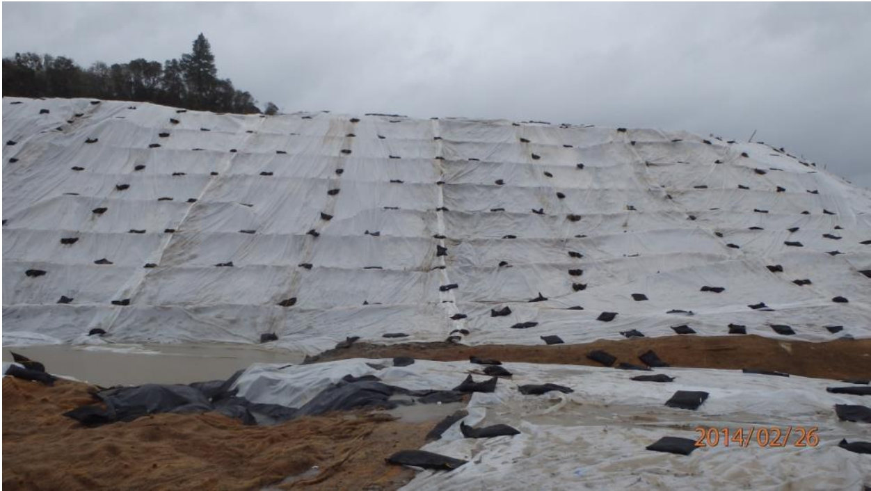
Corrective Action Photo 5E: Looking west at the U2-Line near the inlet to Drainage System 23
