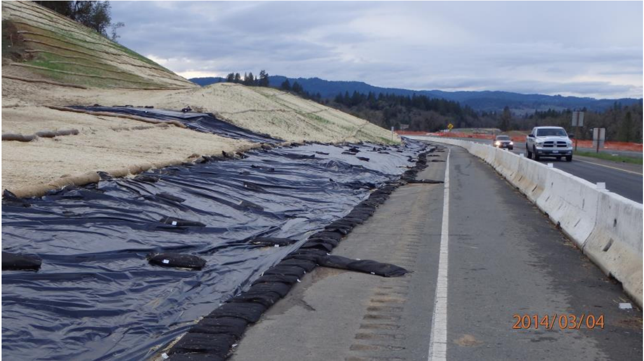
Corrective Action Photo 4A: DSA was stabilized with straw and plastic cover has been installed to convey water along the toe of slope to the drainage inlet. Looking north along Highway 101 at the base of the U1-Line
