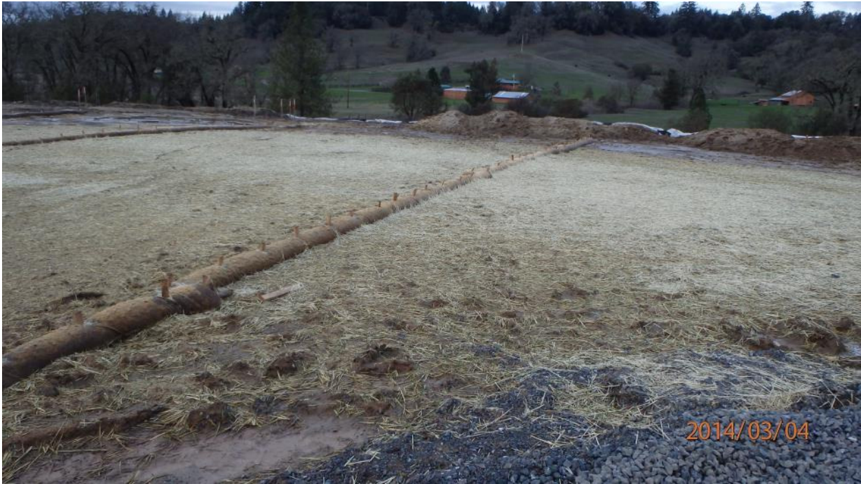
Corrective Action Photo 5D: Straw blown to cover DSA above the U2-Line
