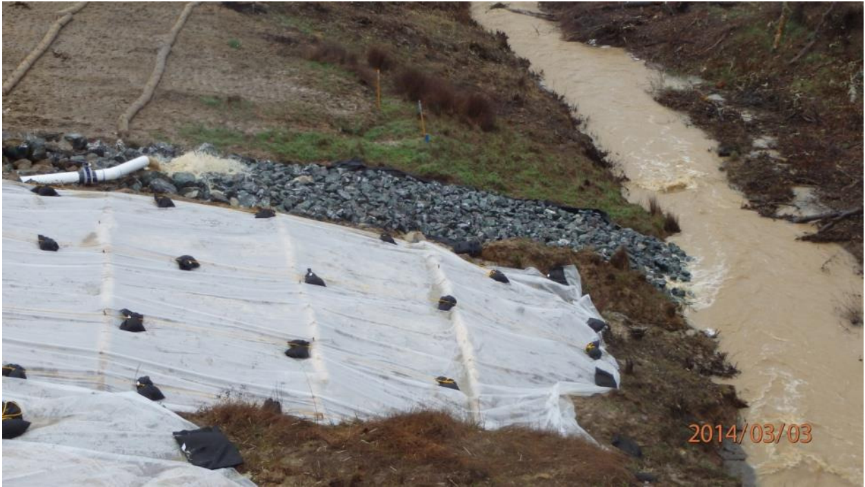
Corrective Action Photo 9A: Looking west along South Haehl Creek at Drainage System 27. RSP has been repositioned and a gravel bag berm has been installed to eliminate water bypassing the drainage
