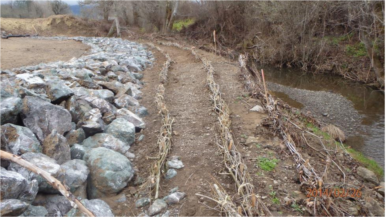
Additional Corrective Action Photo 4: Willow Wattles installed at Drainage System 51 at Baechtel Creek
