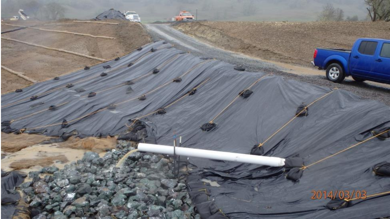
Corrective Action Photo 7C: Looking north from the intersection of the H-Line and the winter access road at the South Haehl Interchange
