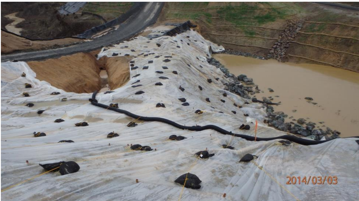
Corrective Action Photo 1B: View from top of Bridge Number 10-0129 RL Northbound Abutment 1. Looking north into South Haehl Creek and the culvert crossing
