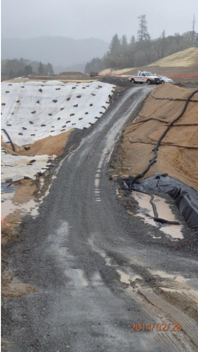
Corrective Action Photo 8A: Looking south at the culvert crossing winter access road at the South Haehl creek. Please refer to Corrective Action Photo 1A and 1D for further corrections
