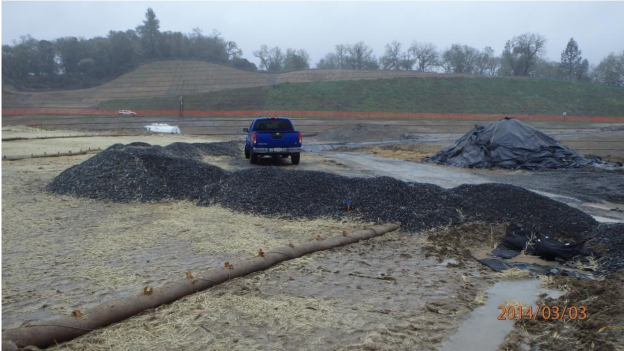
Corrective Action Photo 1A: Top of Bridge Number 10-0129 RL Northbound Abutment 1 with a \frac{3}{4} " gravel berm to divert water into drain under road and straw to cover DSA
