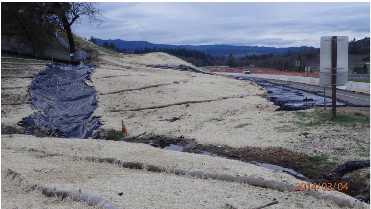
Corrective Action Photo 4B: Looking north along Highway 101 at the base of the U1-Line near the inlet for Drainage System 7
