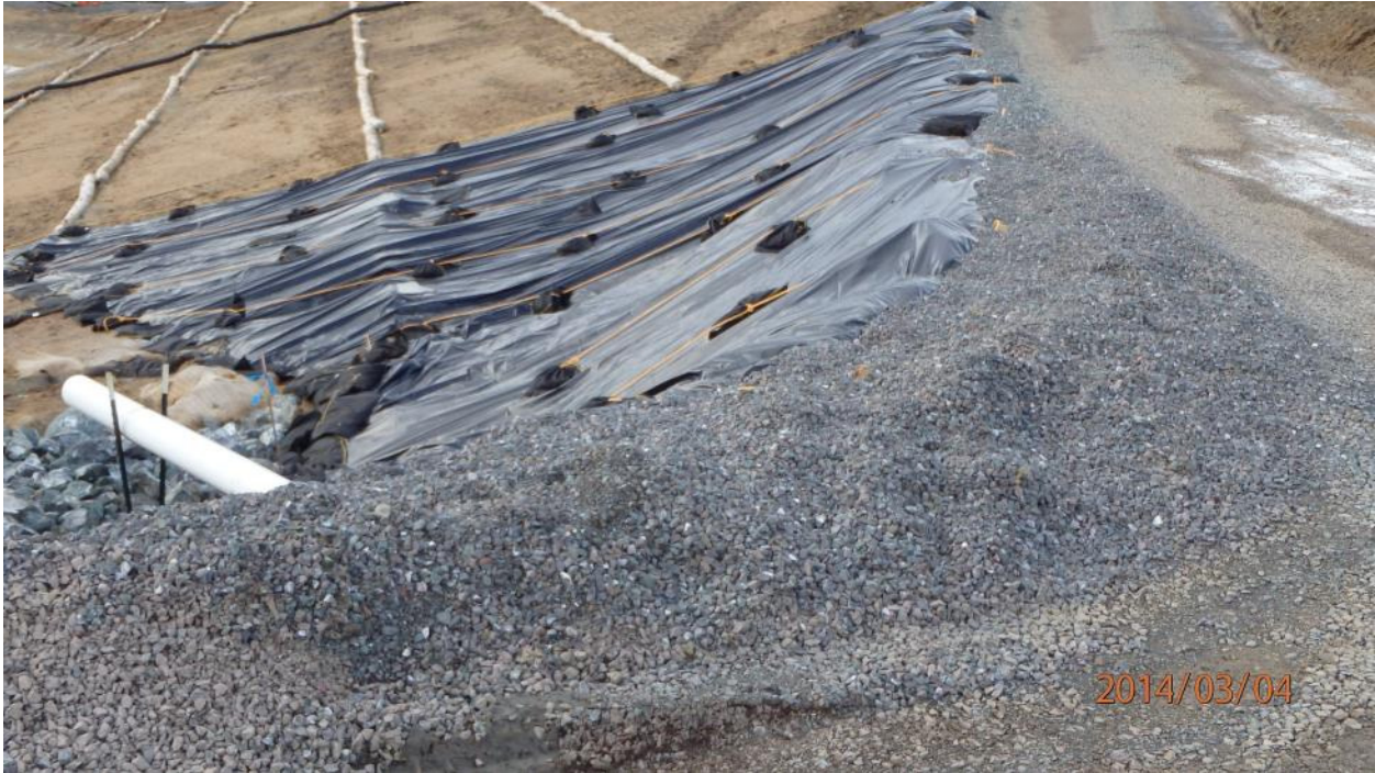
Corrective Action Photo 7A: Pictured is the same location in the NOV Attachment A Photo 7 with a ¾" gravel berm, temporary plastic cover and a drainage pipe installed. Looking north from the intersection of the H-Line and the winter access road at the South Haehl Interchange
