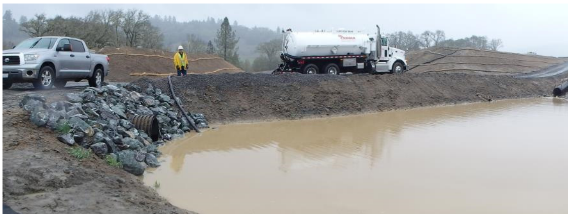
Corrective Action Photo 2A: Pumping water out of the Haehl Creek Interchange basins at the H-Line and winter access road intersection
