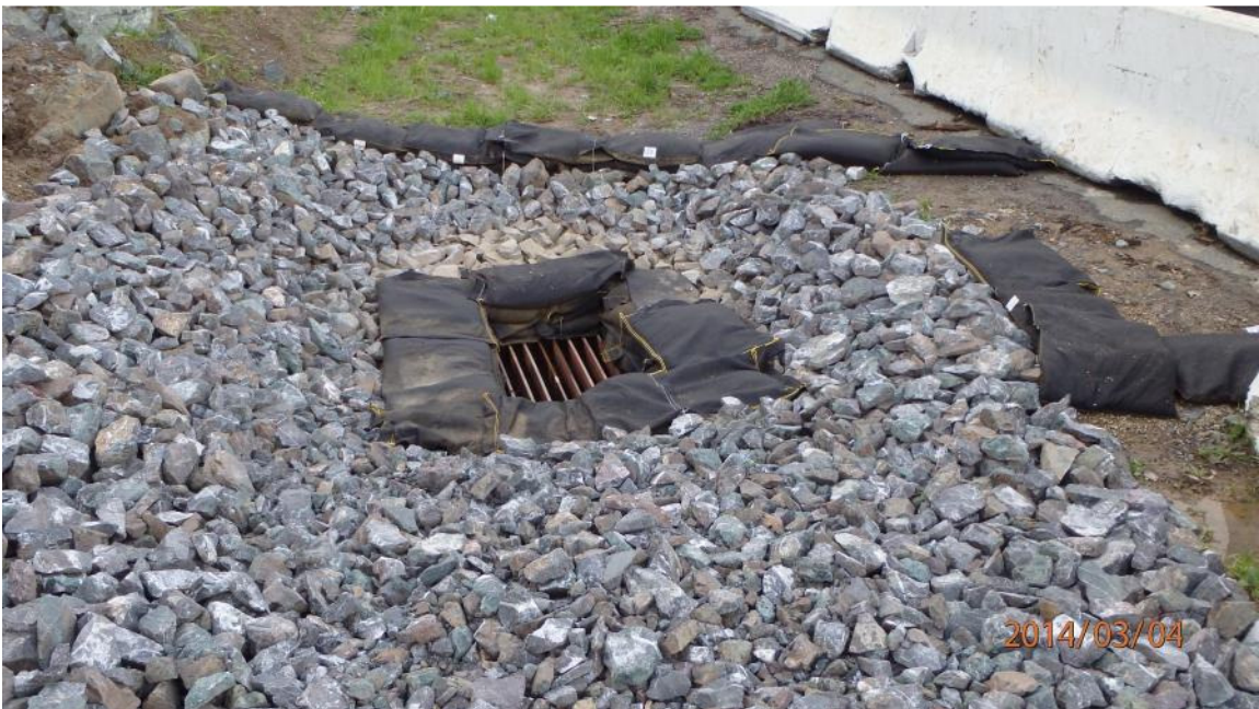
Corrective Action Photo 6B: Looking north along Highway 101 at the base of the U1-Line
