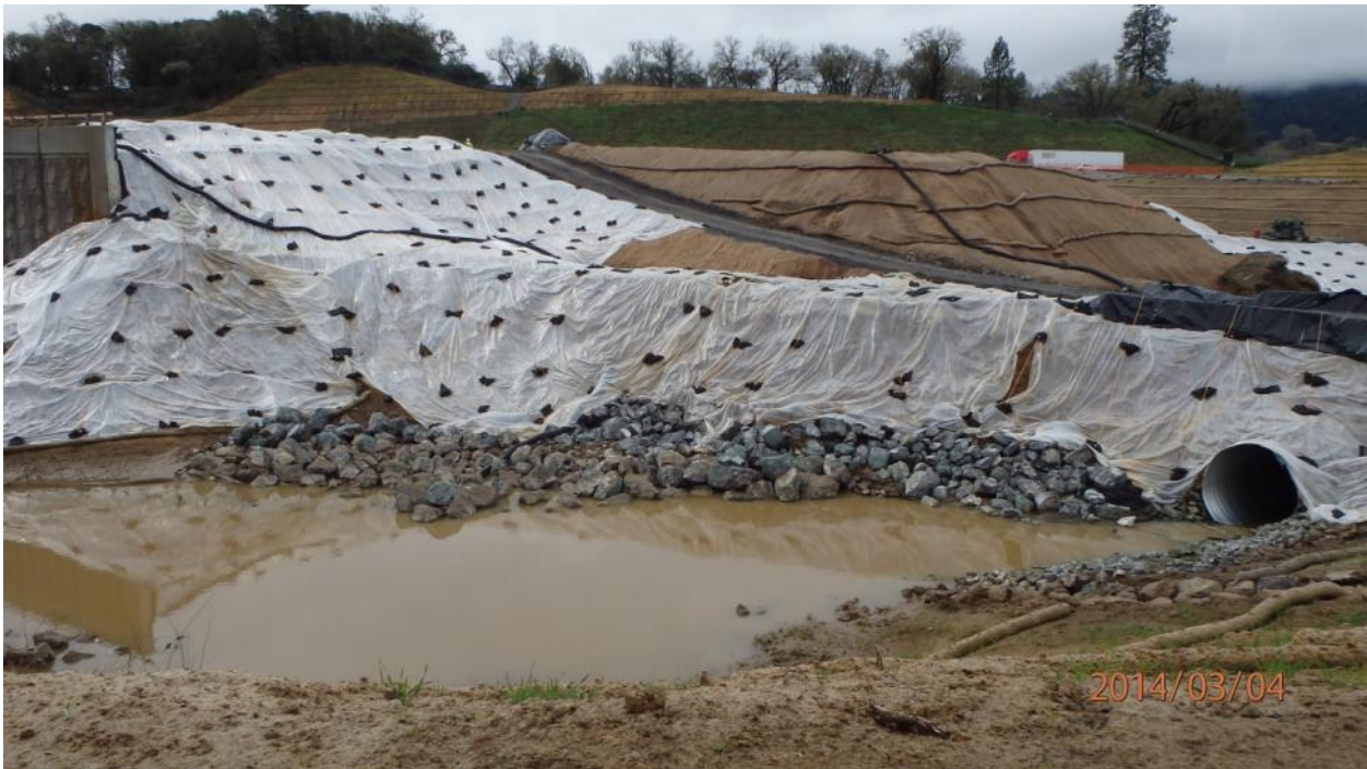
Corrective Action Photo 1C: Looking southwest at the culvert crossing and Bridge Number 10-0129 RL with filter fabric and ¼ ton RSP stabilizing the toe of slope
