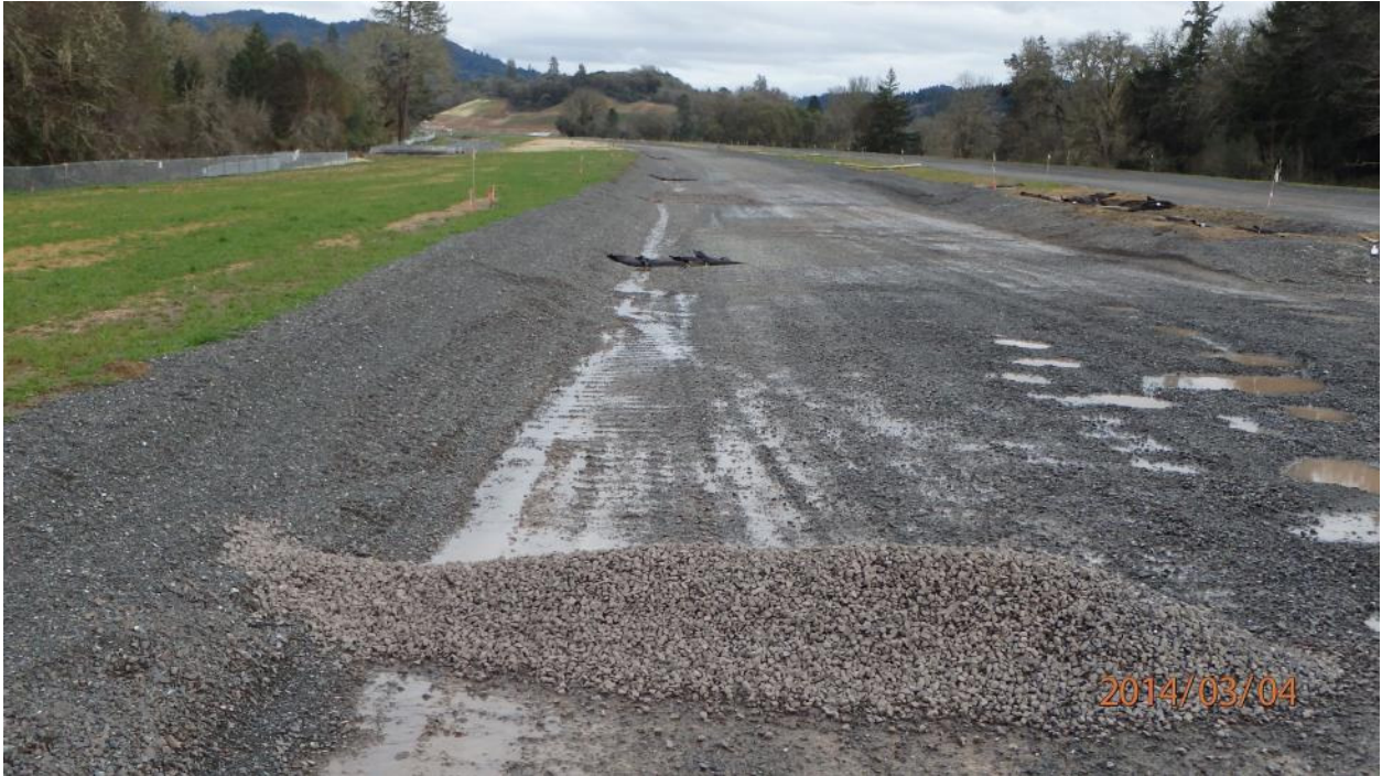
Additional Corrective Action Photo 2: Looking south at the AN-Line with gravel bars and gravel bag check dams. Photo at Station 36+40
