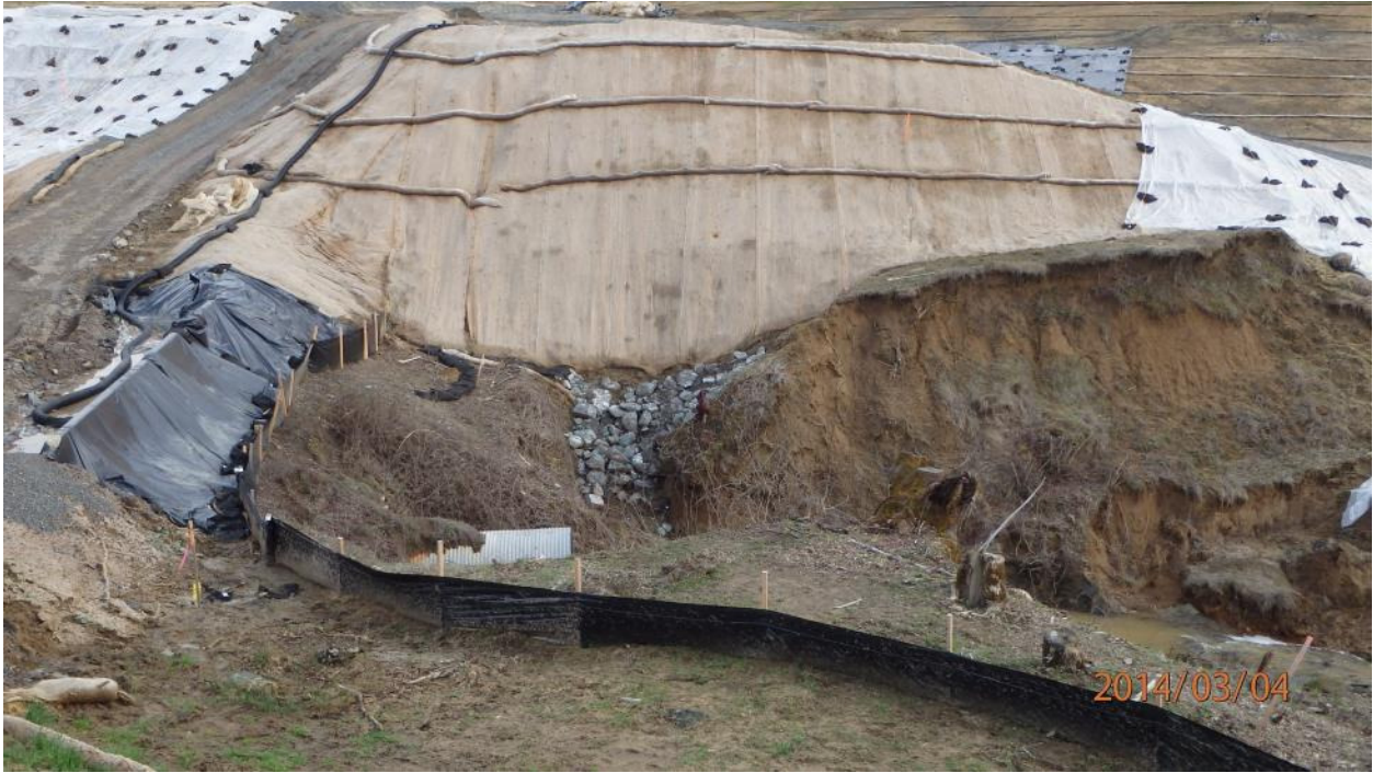
Corrective Action Photo 3A: Looking south at the southbound Bridge Number 10-0129 RL Abutment 1.
