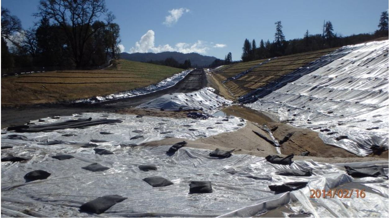
Corrective Action Photo 5A: Looking south at the U2-Line near the inlet to Drainage System 23
