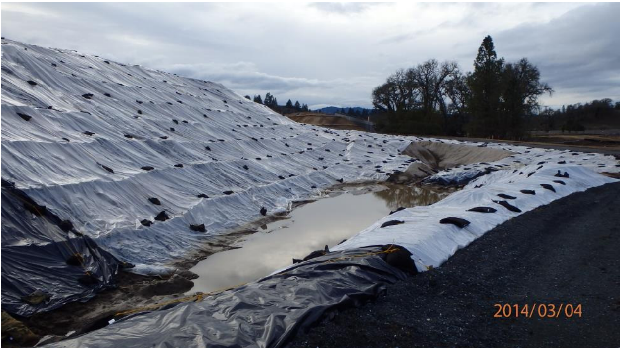
Corrective Action Photo 5B: Looking North along the U2-Line at the inlet to Drainage System 23
