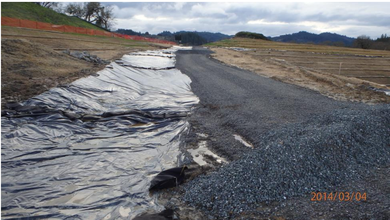
Corrective Action Photo 7C: Looking west at the H-Line with gravel berms and plastic cover conveying water off the road
