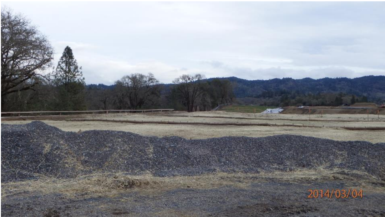
Corrective Action Photo 1D: DSA was stabilized with blown straw at the top of Bridge Number 10-0129 RL Northbound Abutment 1
