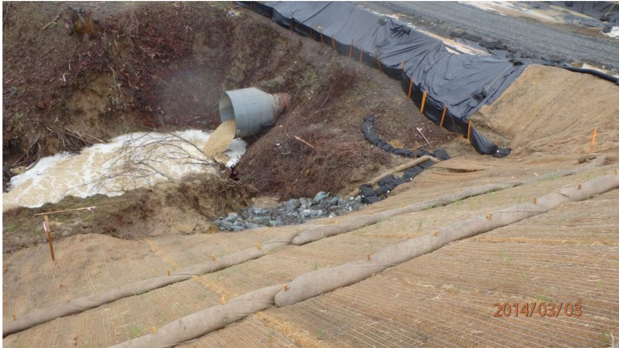
Corrective Action Photo 3C: View from above the southbound Bridge Number 10-0129 RL Abutment 1 at the culvert crossing and South Haehl Creek
