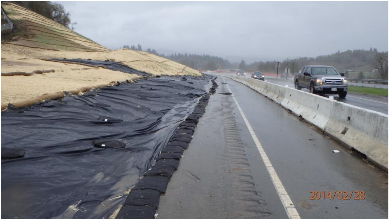
Corrective Action Photo 4C: Looking north along Highway 101 at the base of the U1-Line
