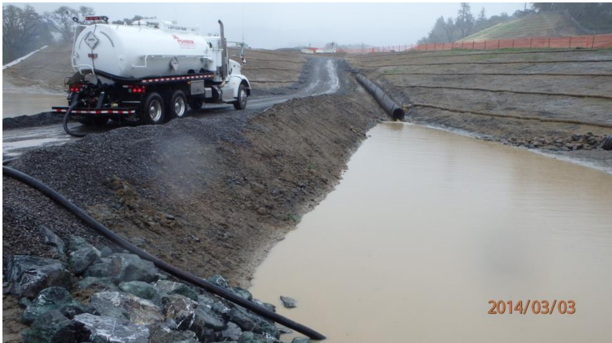
Corrective Action Photo 9B: Pumping water out of the Haehl Creek Interchange basins at the H-Line and winter access road intersection
