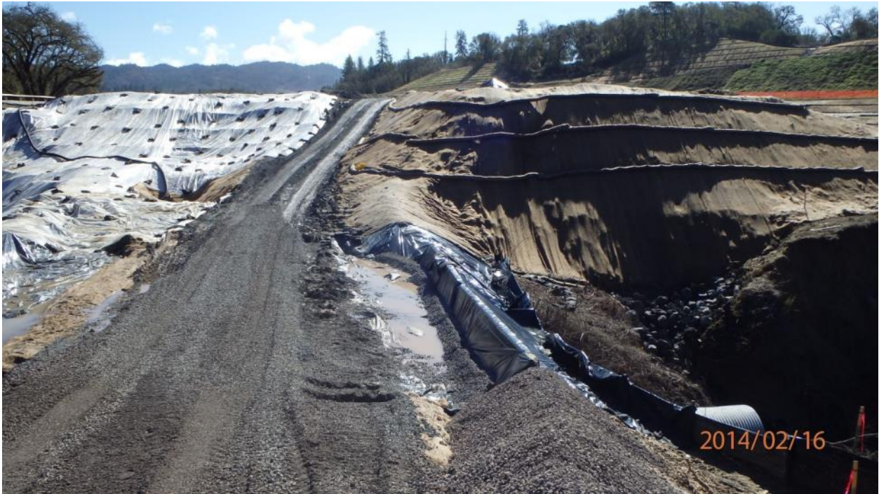
Corrective Action Photo 3B: Looking south at the Bridge Number 10-0129 RL southern abutments
