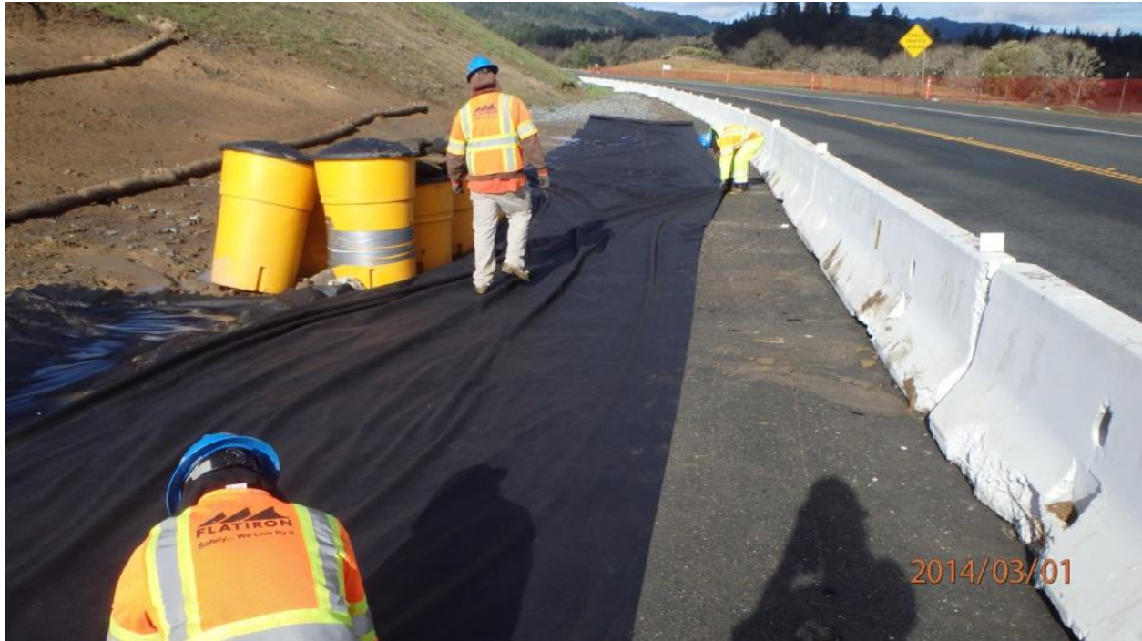
Corrective Action Photo 6C: Crew installing the filter fabric prior to the 3-6" rock installation. Looking north along Highway 101 at the base of the U1-Line
