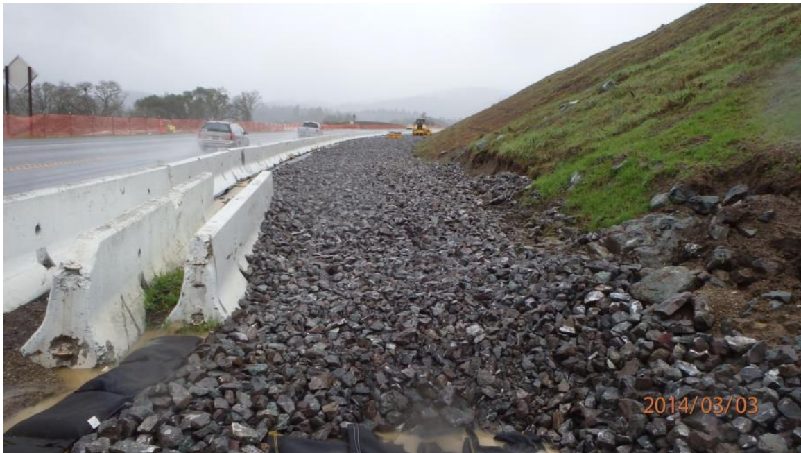
Corrective Action Photo 6D: Drainage inlet has been stabilized with 3-6" drain rock, filter fabric and gravel bags. Looking south along Highway 101 at the base of the U1-Line during the rain
