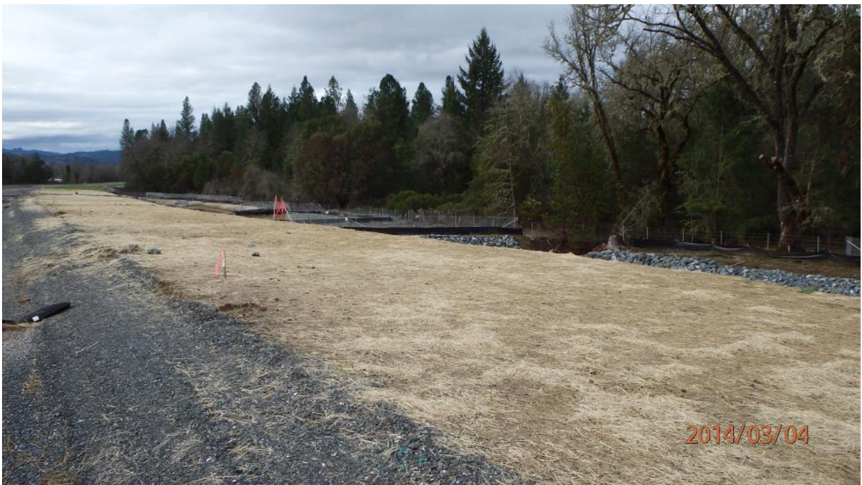
Additional Corrective Action Photo 3: Straw blown to cover DSA at Drainage System 37
