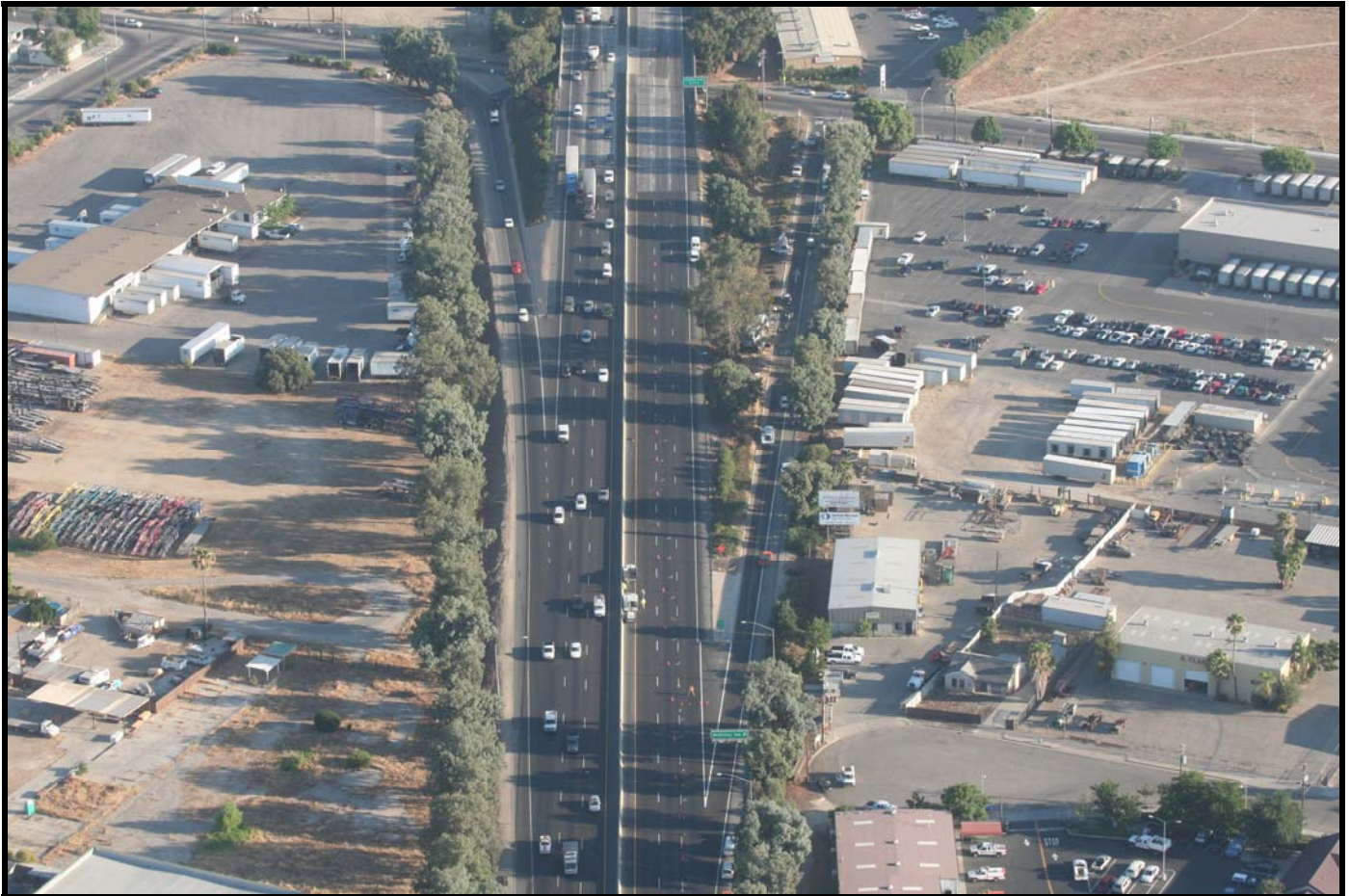
Aerial view of the scene looking north. CF-023-10 07-22-10 DS (45)
