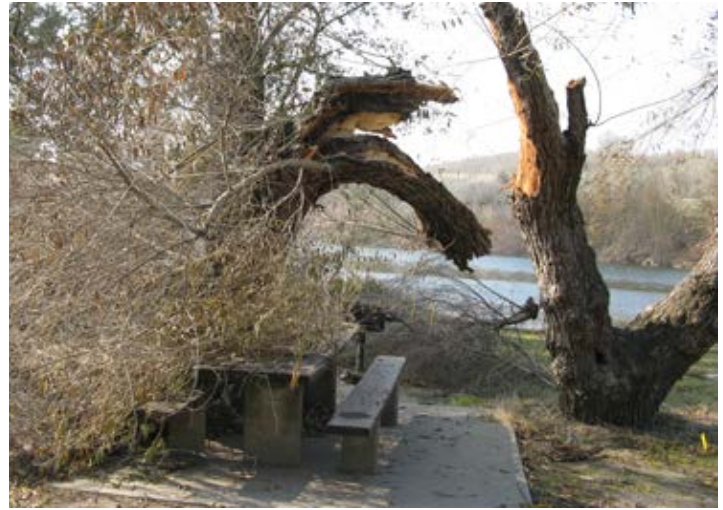
The windstorm also damaged picnic facilities, waterlines and restrooms.
